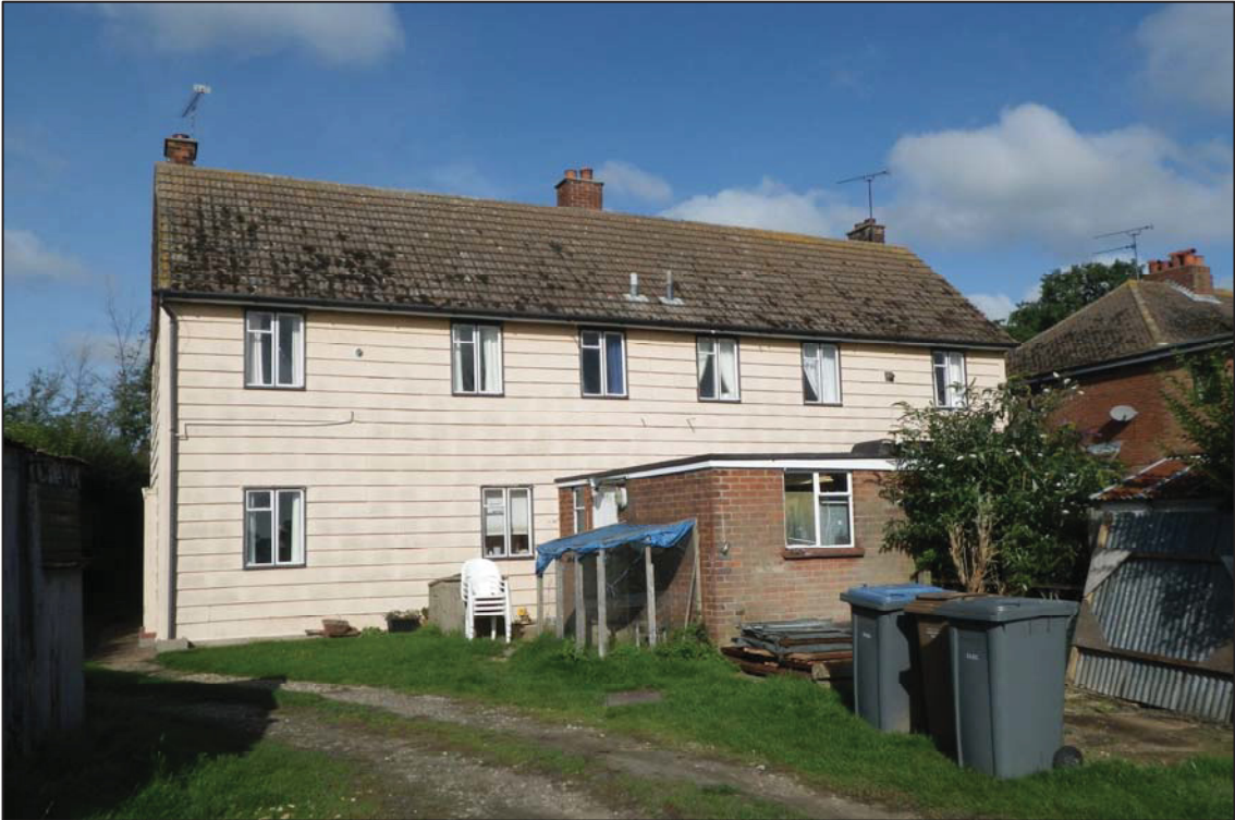
Plate 2. General view of the rear of Nos. 39 and 41 (ref. HTR 67)
