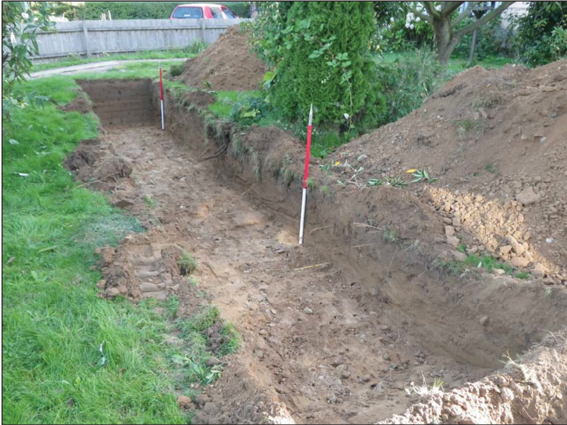
Plate 3. Trench 1, general view (ref. HTR 68)
