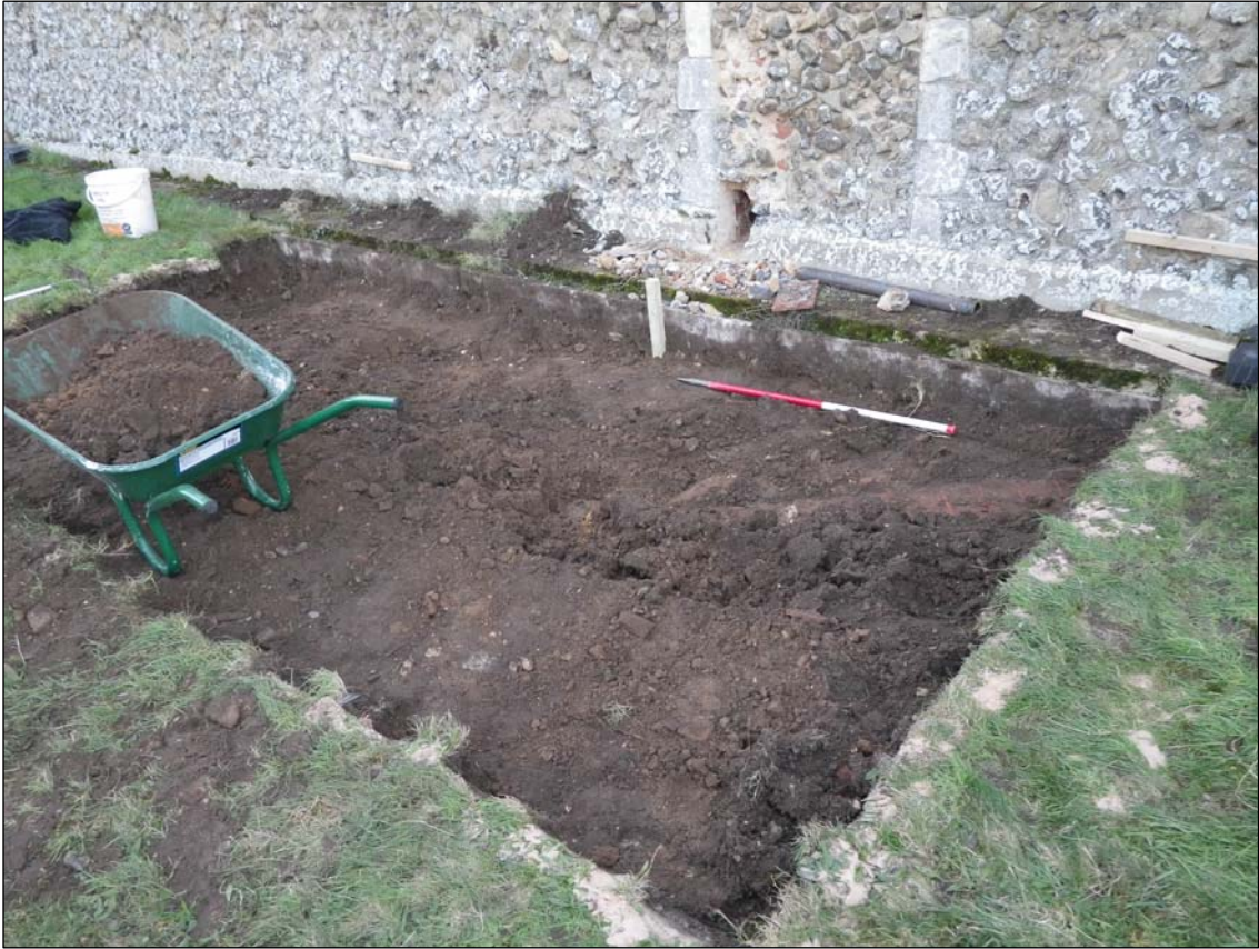
Plate 1. Stripped extension footprint, looking SE
