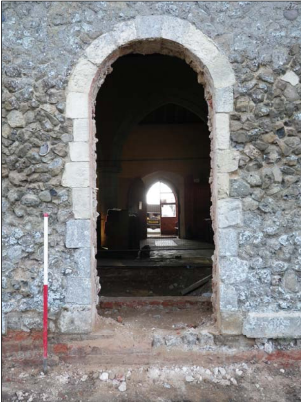
Plate 3. The north doorway, looking S. The worked limestone was recovered from the void just inside the doorway, in front of the red bricks
