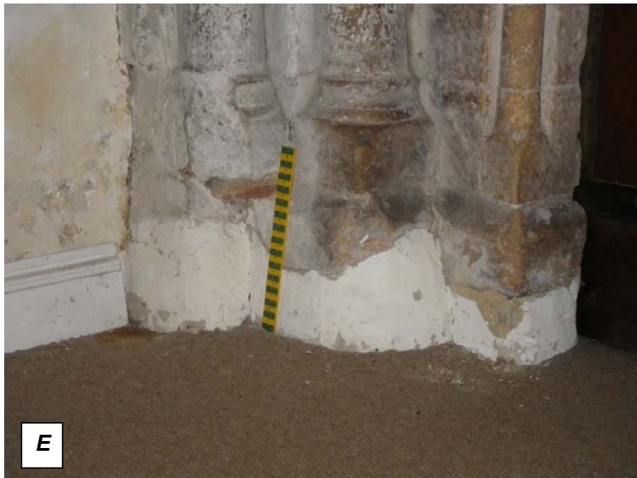
E) Column bases, part of what was once the west and main door of the church which is now enclosed in the 14th century tower. Outside the tower the ground level is higher than this and the west door of the tower is reach by a short flight of steps. .
