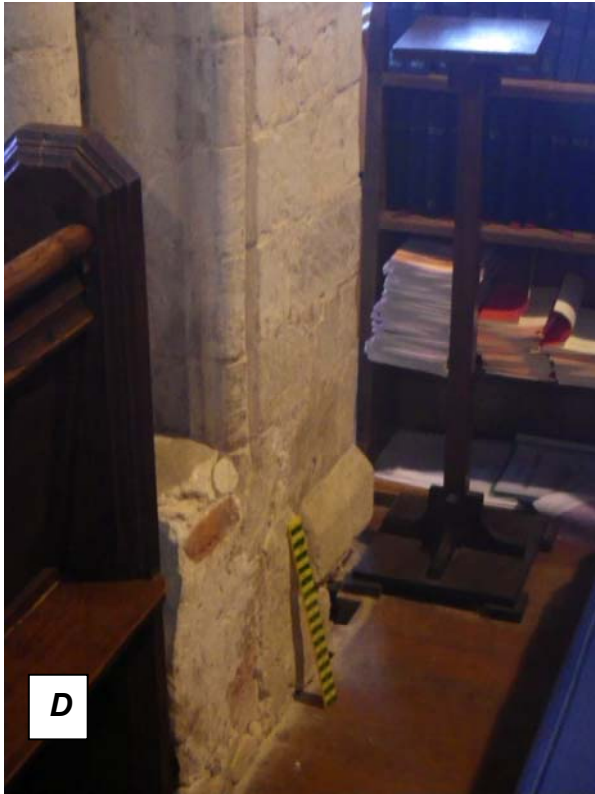
D) Pier base of the Norman arcade illustrating by how much the floor has been lowered.
