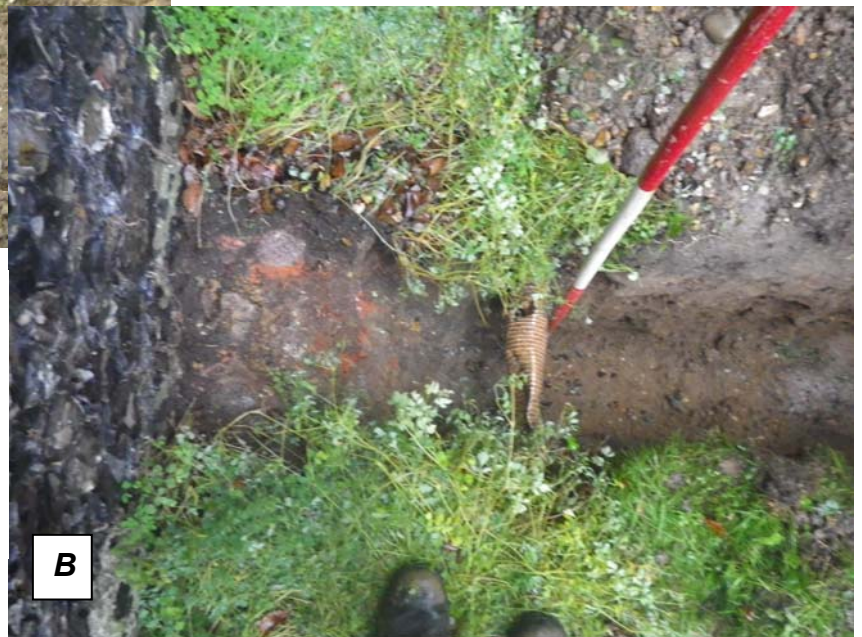
B) Footing seen from above showing how far it projected forward of the wall. The brickwork is a later addition cemented to the top of the medieval flintwork to consolidate the footing.
