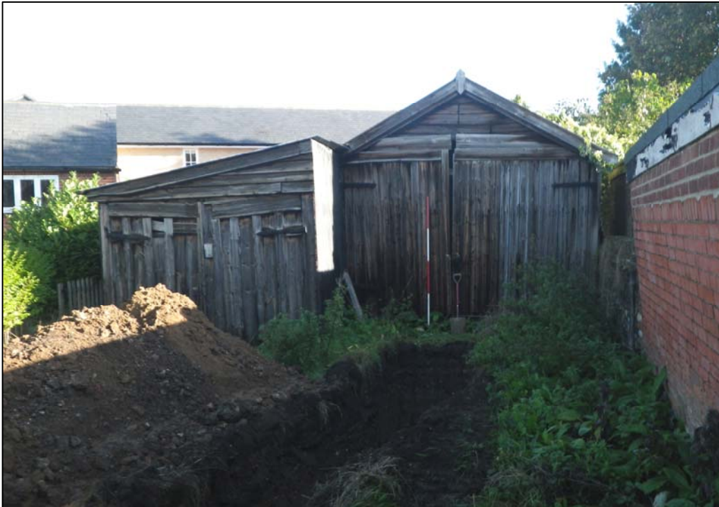
Plate 1. General view of the outhouses to be demolished (ref. HUI 76)
