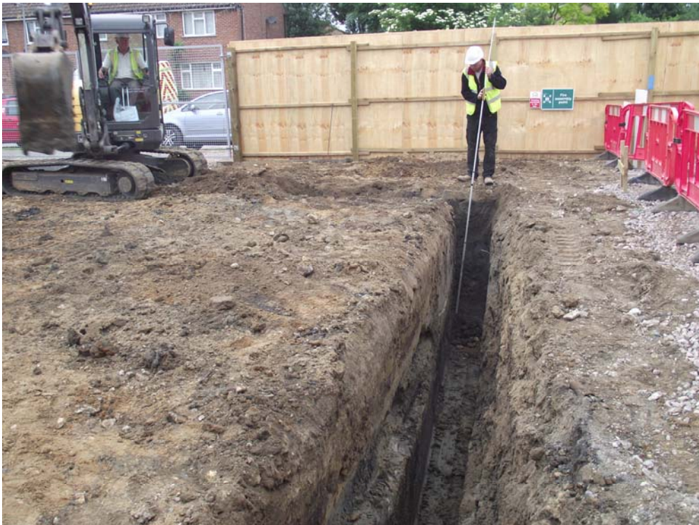
Plate 2. View along footing trench showing depth of deposits, looking north
