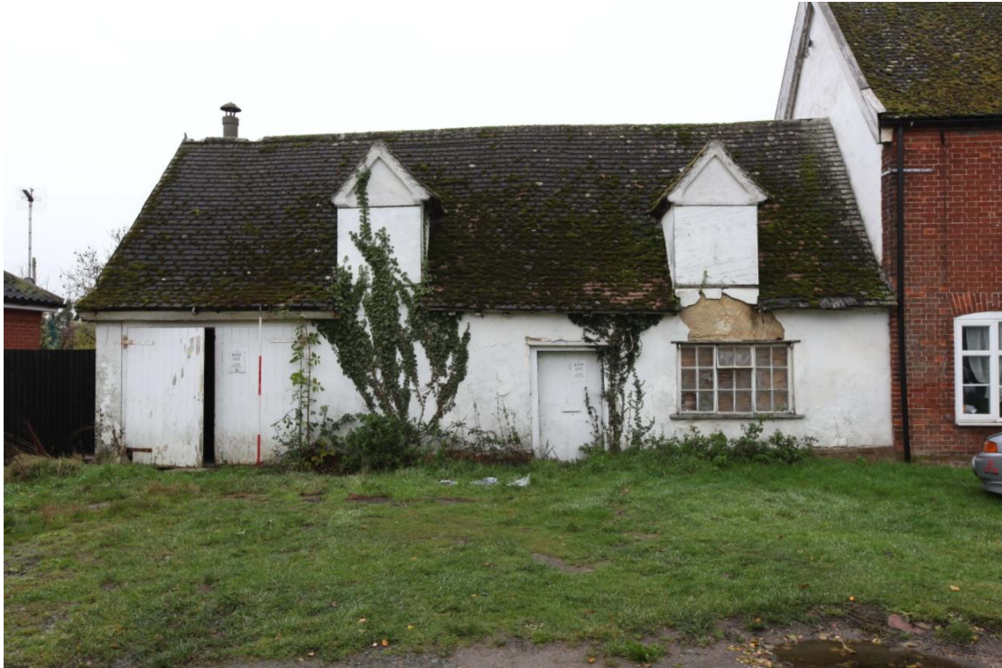
Illus. 3. The eastern facade showing the building's mid-20 th century cement tiles and rendered timber-framed walls. The double doors to the left open into a brick garage (G) that probably replaced a 17 th century extension damaged by the fire of 1963. The diminutive original structure may have formed the dwelling of the potter who is understood to have worked on the site as early as the 16 th century.
