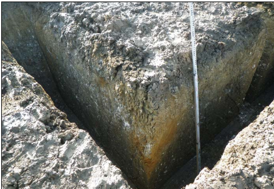
Plate 1. Garage footings (facing south-west)
