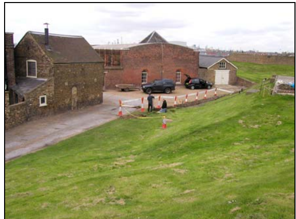
Plate IV: General view of work underway. Camera facing northwest
