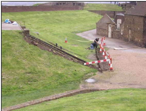
Plate III: General view of work underway. Camera facing southeast
