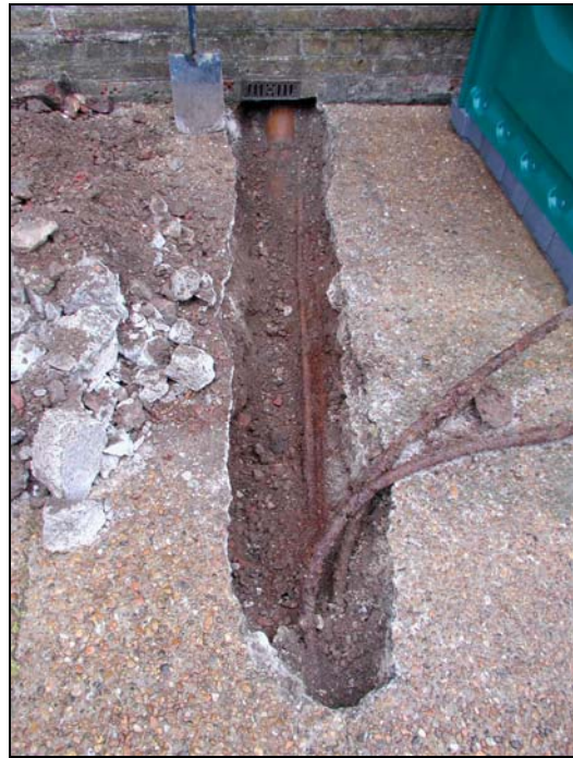
Plate IV: Trenches 1 after excavation
