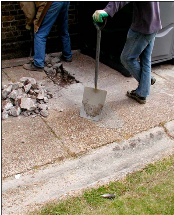
Plate III: Site of Trench 1 Illustrating 'scar' from previous excavation
