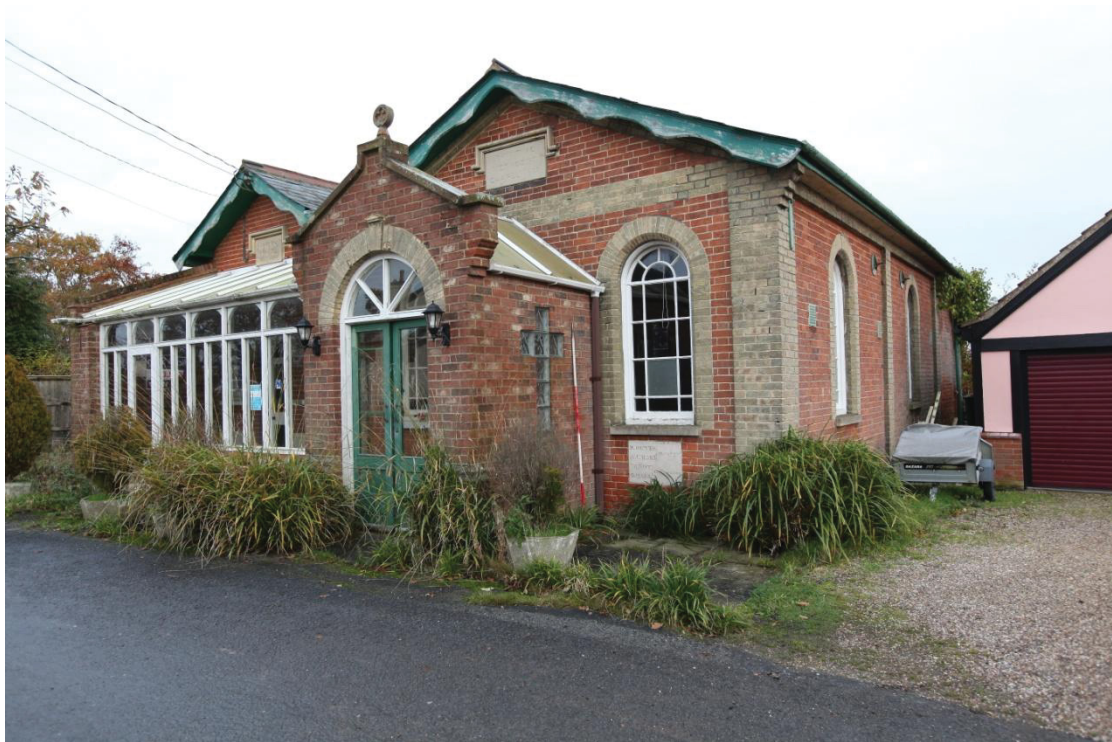
Illus. 2. The exterior of the chapel from the south-west showing its twin gables with the late-20 th century brick porch and glazed lobby extension (1) adjoining the road. Note the glazed cruciform window to the southern side of the porch.
