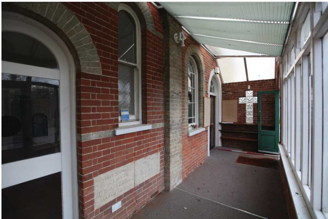
Illus. 6. The interior from the north of the late-20th century entrance lobby and porch (1) showing the facade of the original hall (2) in the rear to the left and the matching Sunday School on the left. Both doors are modern.
