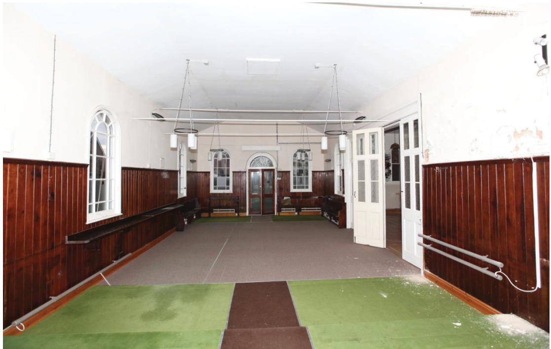
Illus. 8. The interior of the original hall of 1873 (2) from the raised dais to the east showing its stained pine wainscot panelling with the 20 th century glazed doors to the Sunday School extension on the right and the central western entrance in the rear.
