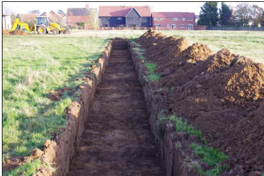
Plate 5. General view of Trench 5, looking east
