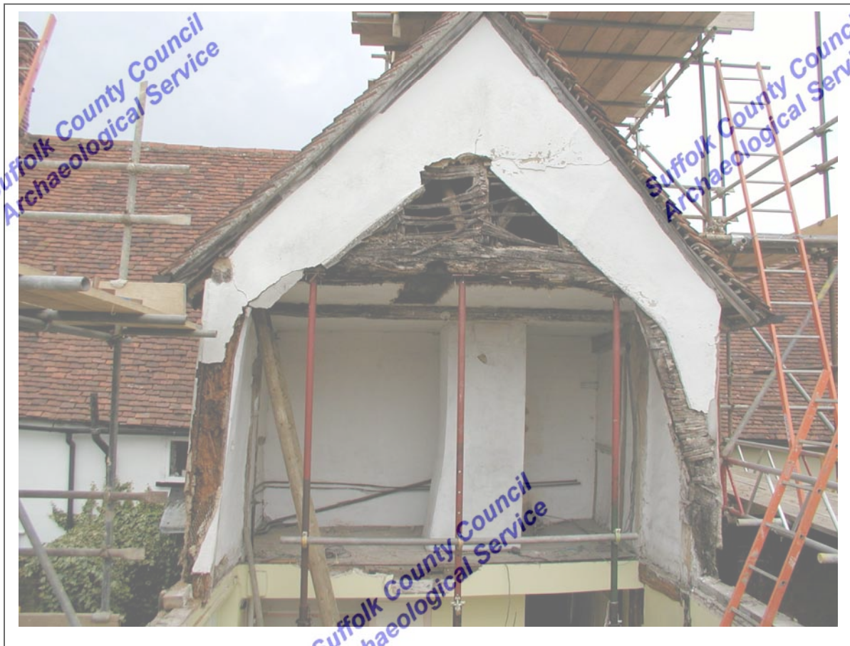
Fig. 8 Western gable-end of the southern cross-wing (looking east)
