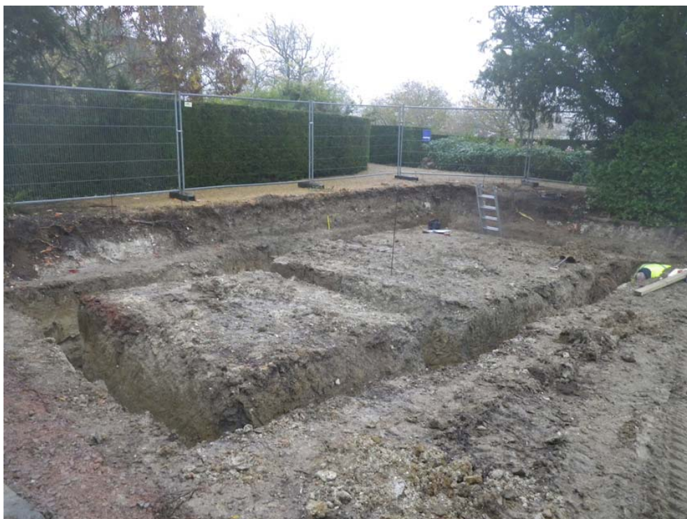
Plate 4. Strip footing for the changing rooms at the north end of the development area looking north towards the hall. The path beyond the far corner of the site is on the line of the medieval driveway and approach to the bridge through the break in the hedge. The area has been reduced by the partial removal of the redeposited clay which can be seen in section on the edge of the site. The 'reduced-dig' level is close to but still above the medieval ground level which is considerably lower than the access to the bridge. Does this imply that the driveway was on a raised causeway at this point? The driveway ditch which crosses this area is beneath the clay.
