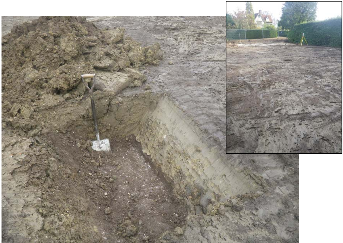
Plate 3. Thick layer of compacted redeposited clay covering the entire development area photographed following the removal of a thin topsoil layer. The clay, the result of dumping either from moat dredging or the excavation of a previous swimming pool alongside the development area, was relatively clean and contained only a few small fragments of brick/tile. The former ground surface can be seen in the main picture at the bottom of the test hole.
