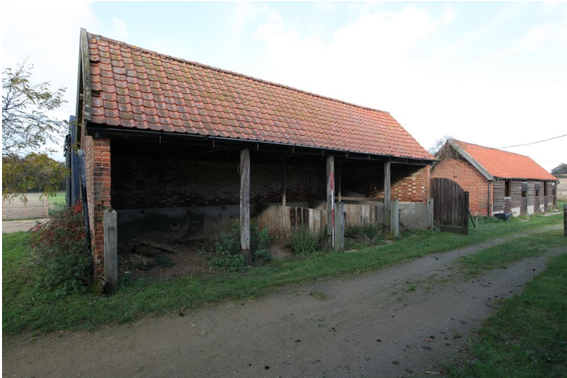
Illus. 3. The open-sided southern exterior of the late-19 th century western shelter-shed (2) which initially served the stable (4) immediately opposite. The contemporary eastern shelter-shed (6) to the right was converted into a stable in the late-20 th century. The parish boundary between Iken and Sudbourne runs along the track in the foreground.
