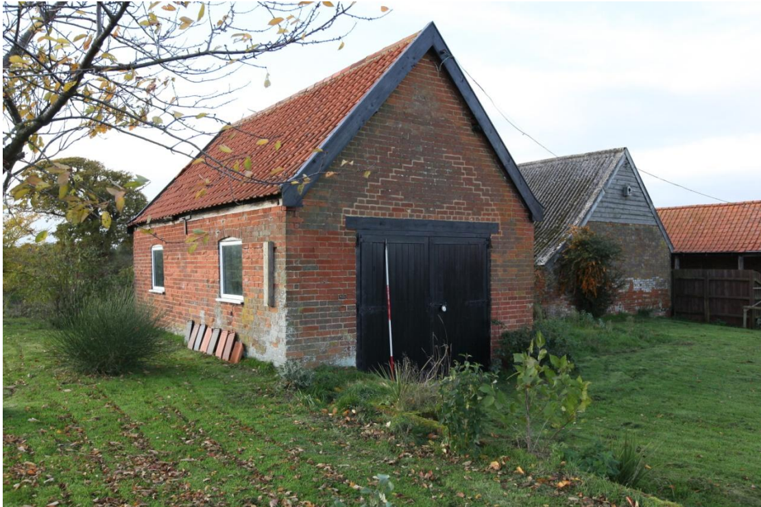
Illus. 5. The late-19 th century brick vehicle shed (5) from the east showing the replaced doors occupying its original gable entrance and two original window apertures in the southern elevation. There is evidence of a narrow original door in the opposite western gable (now converted into a window). The stable (4) with its integral southern lean-to is visible to the right.
