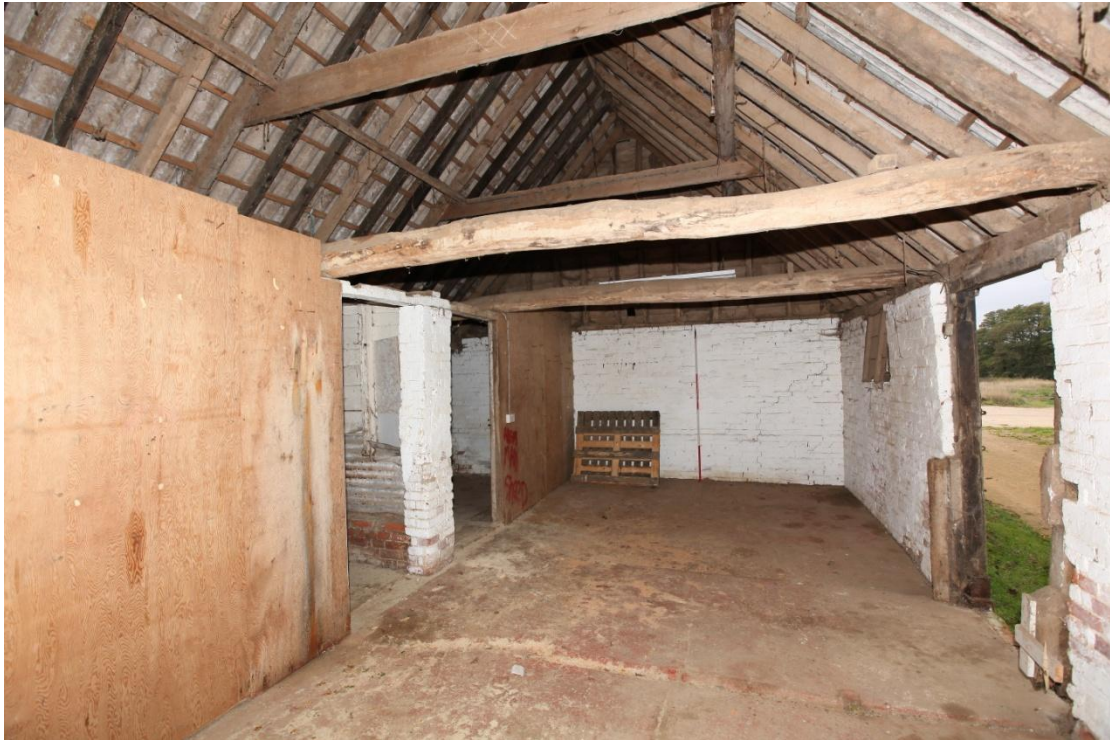
Illus. 9. The interior of the 19 th century stable (4) from the east, showing its central entrance to the right and the twin central doors opening into the two compartments of the integral rear lean-to on the left. The roof was rebuilt in 1923 as dated by an inscription on the further of the two roof collars shown here. The horses were presumably stalled against the gables, although no evidence survives, with the lean-to containing a tack room and chaff box.
