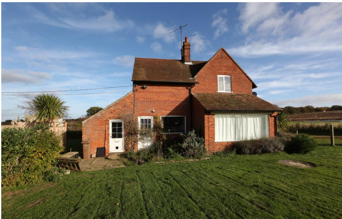
Illus. 12. The early-20 th century farmhouse (7) from the west. The northern lean-to on the left is an original feature but that to the right is a late-20 th century addition. A pair of mill stones serves as door steps and may have been used to grind animal feed on the farm. The present house appears on the Ordnance Survey of 1927 but not that of 1904 and appears to date from circa 1910. It may, however, be contemporary with the re-roofing of the stable (4) in 1923.
