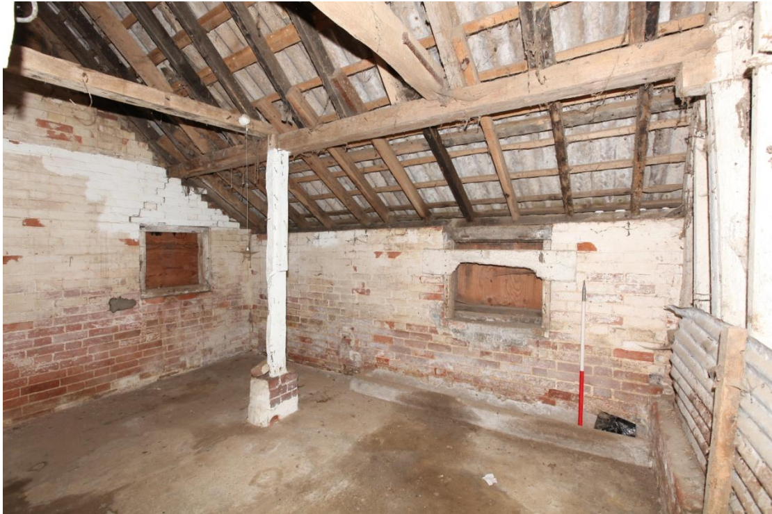
Illus. 11. The interior from the north-west of the easternmost lean-to compartment of the 19 th century stable (4) showing two original windows or loading hatches with a late-20 th century concrete cattle trough. Part of this space may have served as a chaff box.
