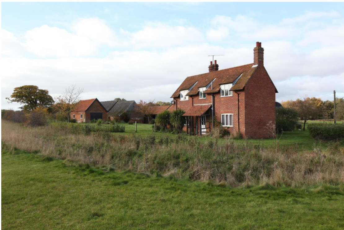
Illus. 2. A general view from the south-east showing the early-20 th century red-brick farmhouse (7) to the right with the late-19 th century vehicle shed (5) to the left and the mid-19 th century stable (4) in the centre.
