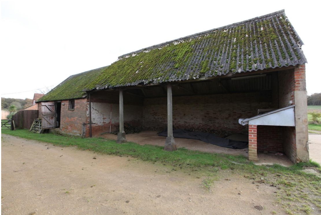
Illus. 7. The 19 th century cart lodge (2) at the entrance to the site as viewed from the north-west and showing its original open arcade with the contemporary or slightly earlier stable (4) on the left.
