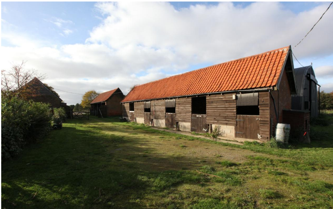
Illus. 4. The late-19 th century eastern shelter-shed (6) seen from the east, with the Nissen hut (1) in the rear to the right and the stable (4) and western shelter-shed (2) on the left. The buildings to the north (right) of the track are in Iken but the farmhouse and other structures lie in Sudbourne parish. The southern elevation of the shelter-shed was originally open to match its western counterpart but was enclosed in the late-20 th century to form a stable consisting of five loose boxes.
