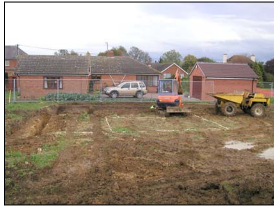
Plate II: Excavation of Plot 2
