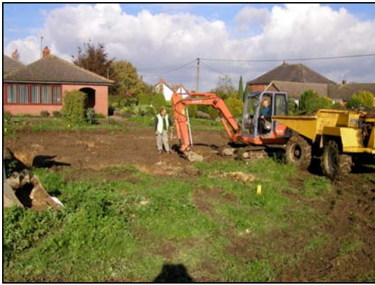
Plate I: Excavation of Plot 1
