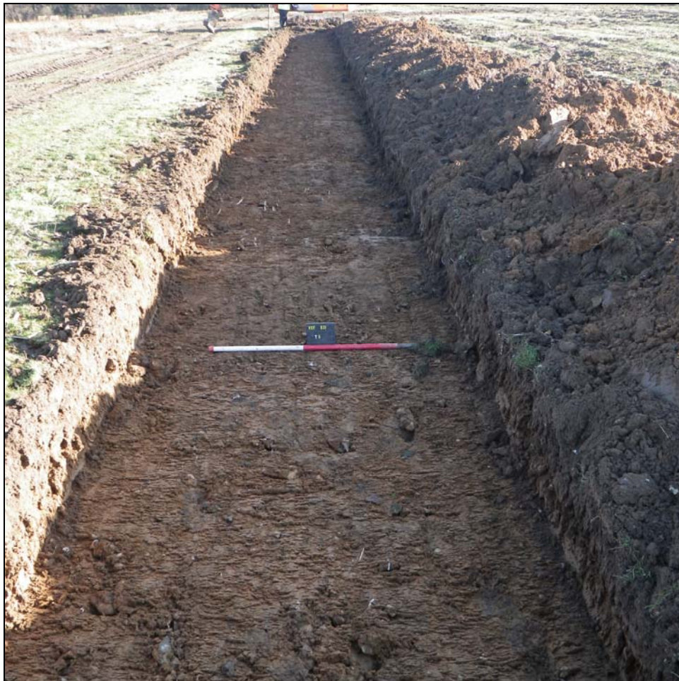
Plate 3. Trench 5, facing east (1m scale)
