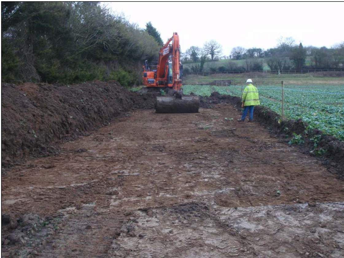
Plate 1. Topsoil stripping of the easement
