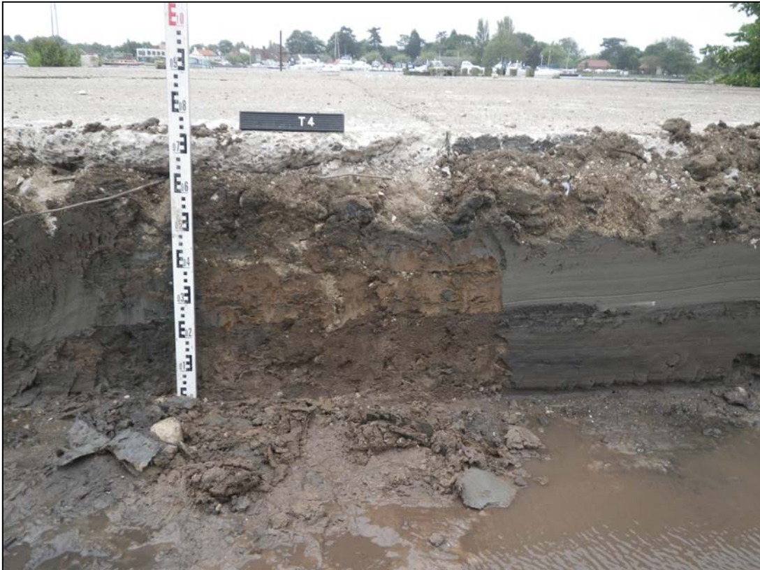
Plate 7. Trench 4, camera facing south (ref. HWZ 51)
