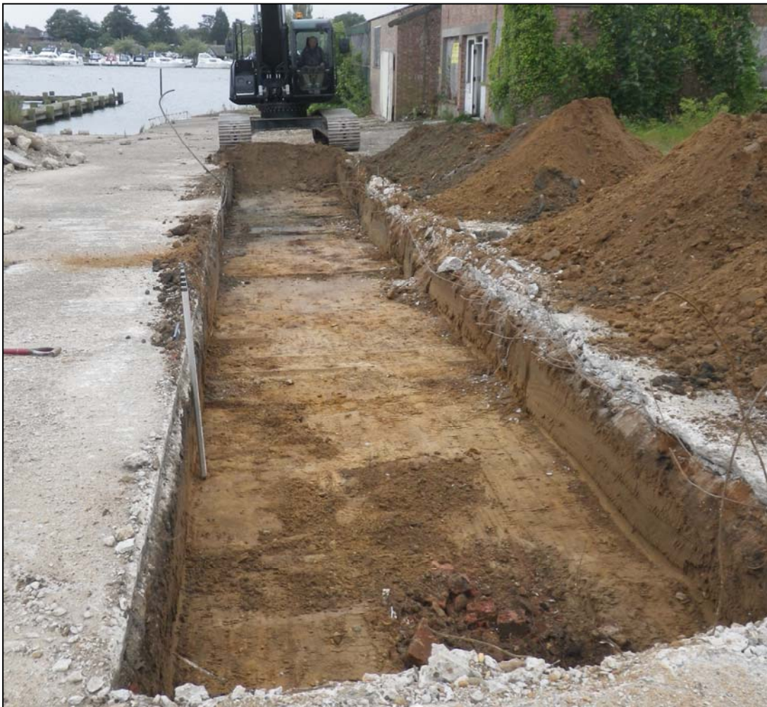
Plate 10. Trench 5, camera facing south (ref. HWZ 56)
