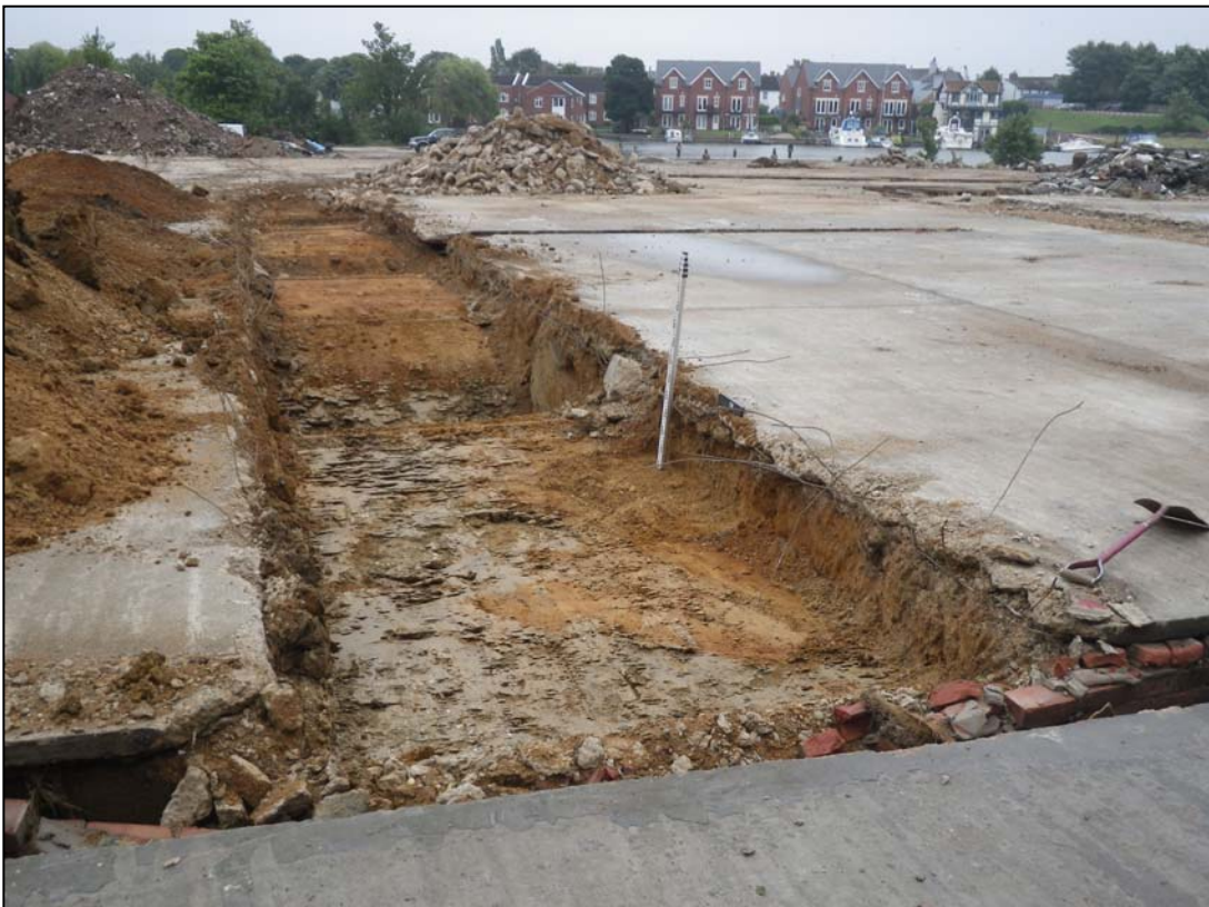
Plate 16. Trench 8, camera facing east (ref. HWZ 64)
