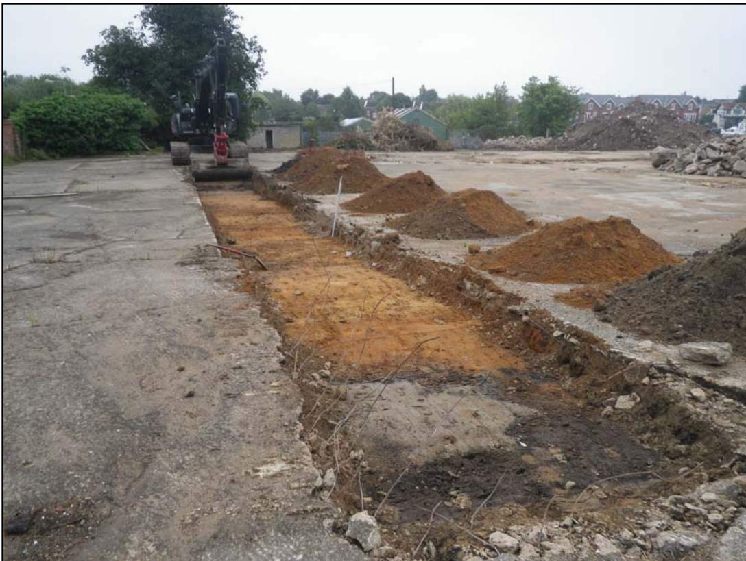
Plate 20. Trench 10, camera facing east (ref. HWZ 68)
