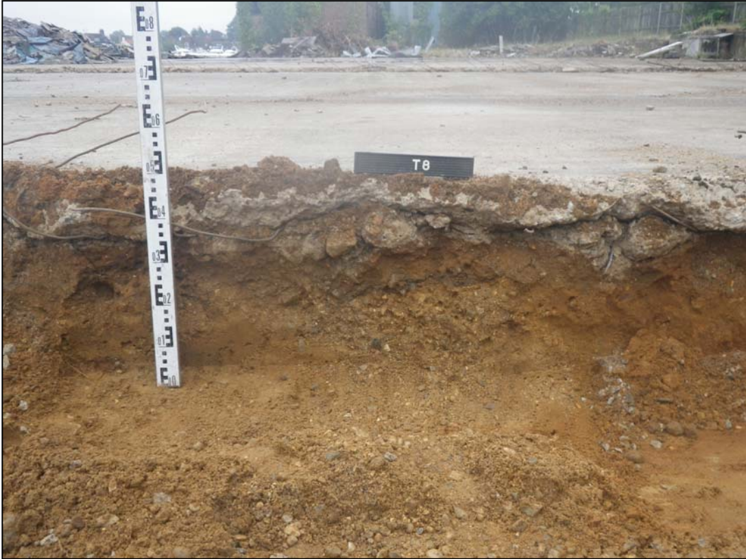
Plate 15. Trench 8, camera facing south (ref. HWZ 63)
