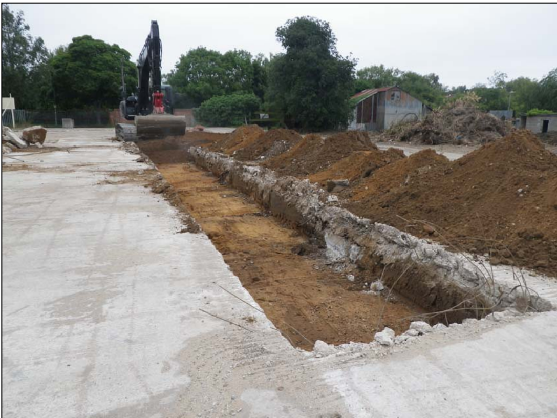
Plate 14. Trench 7, camera facing north (ref. HWZ 62)
