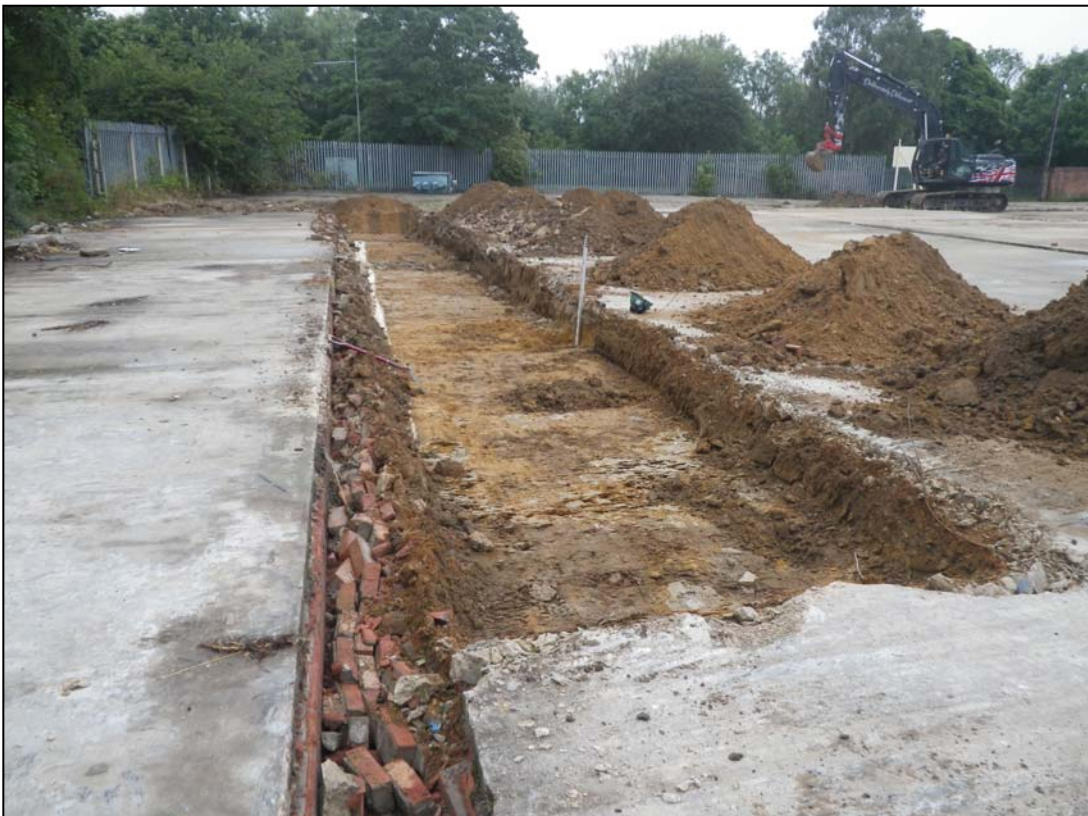
Plate 18. Trench 9, camera facing north (ref. HWZ 66)
