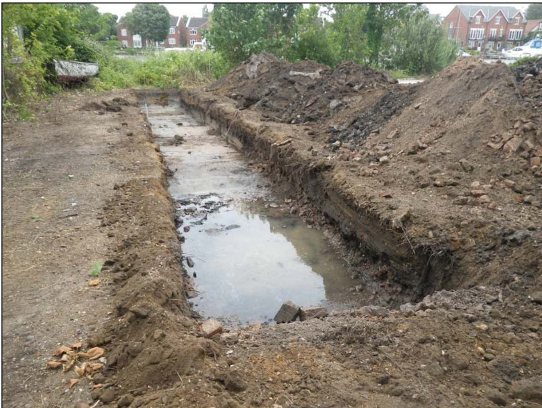
Plate 4. Trench 2, camera facing east (ref. HWZ 48)
