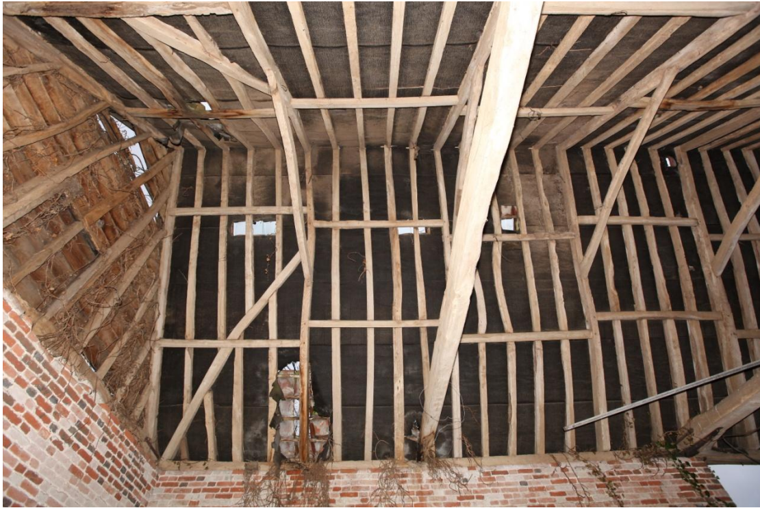
Illus. 11. The unusually intact staggered butt-purlin roof structure in the eastern half of the barn, looking south, with original primary braces interrupting the rafters in the end-bay to the left. The roof of the western half is identical.
