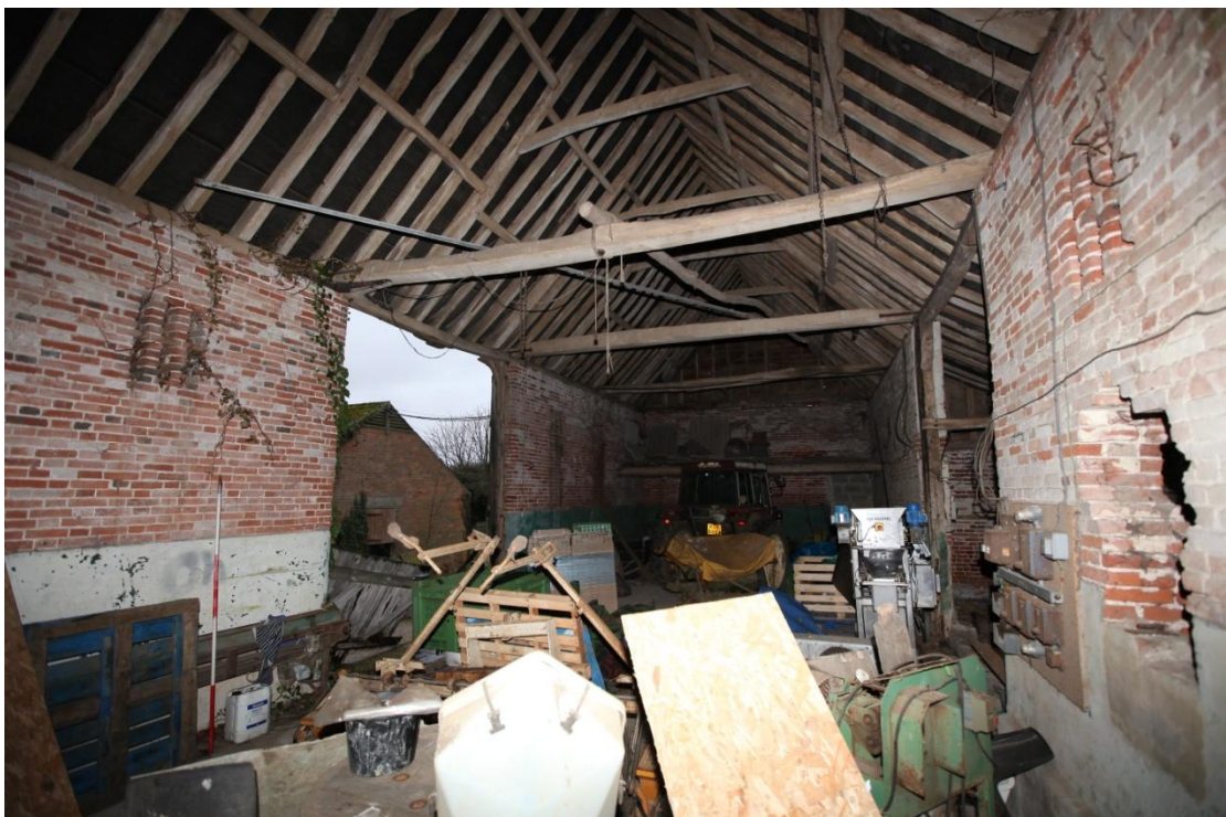
Illus. 8. The interior from the east showing the original central entrance to the threshing bay on the left and the later aperture to the porch on the right.
