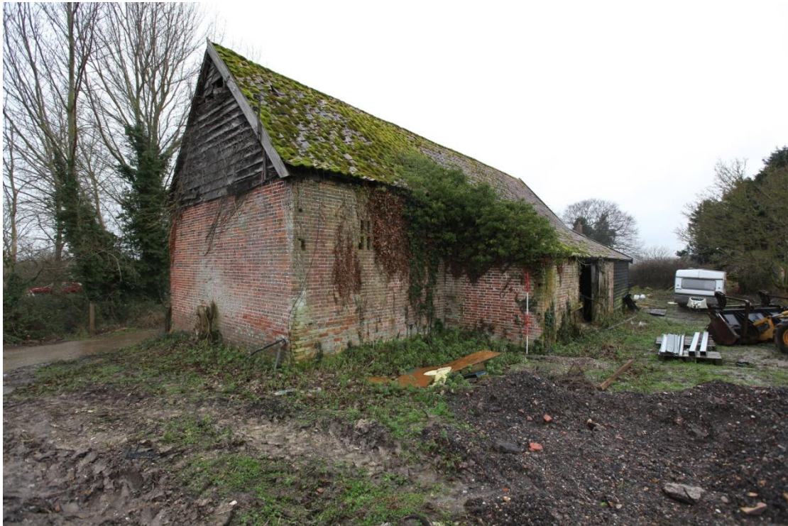
Illus. 4. The barn from the north-east showing the original weatherboarded studwork of the roof gable. An aperture in the brickwork of the northern elevation is likely to have secured the tie-beam of a second weatherboarded lean-to shed as depicted on the historic Ordnance Surveys but subsequently demolished.
