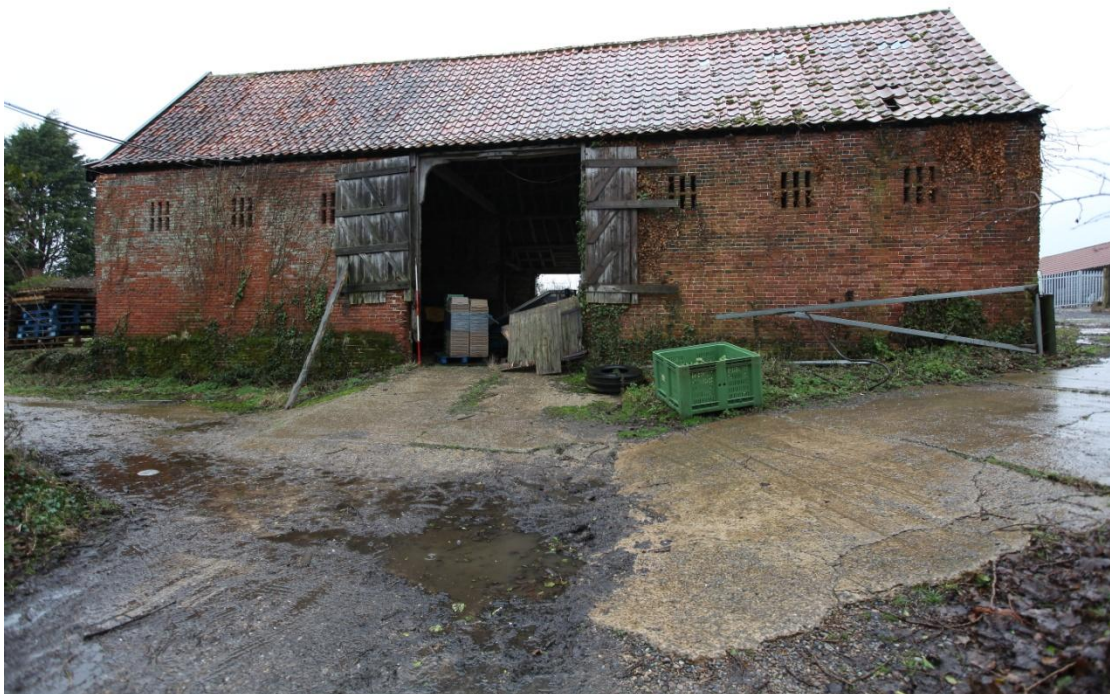
Illus. 2. The barn's well-preserved southern facade with three groups of original ventilation loops on each side of the central entrance. The fragmentary half-hung doors are replacements of the late-19 th or early-20 th century.
