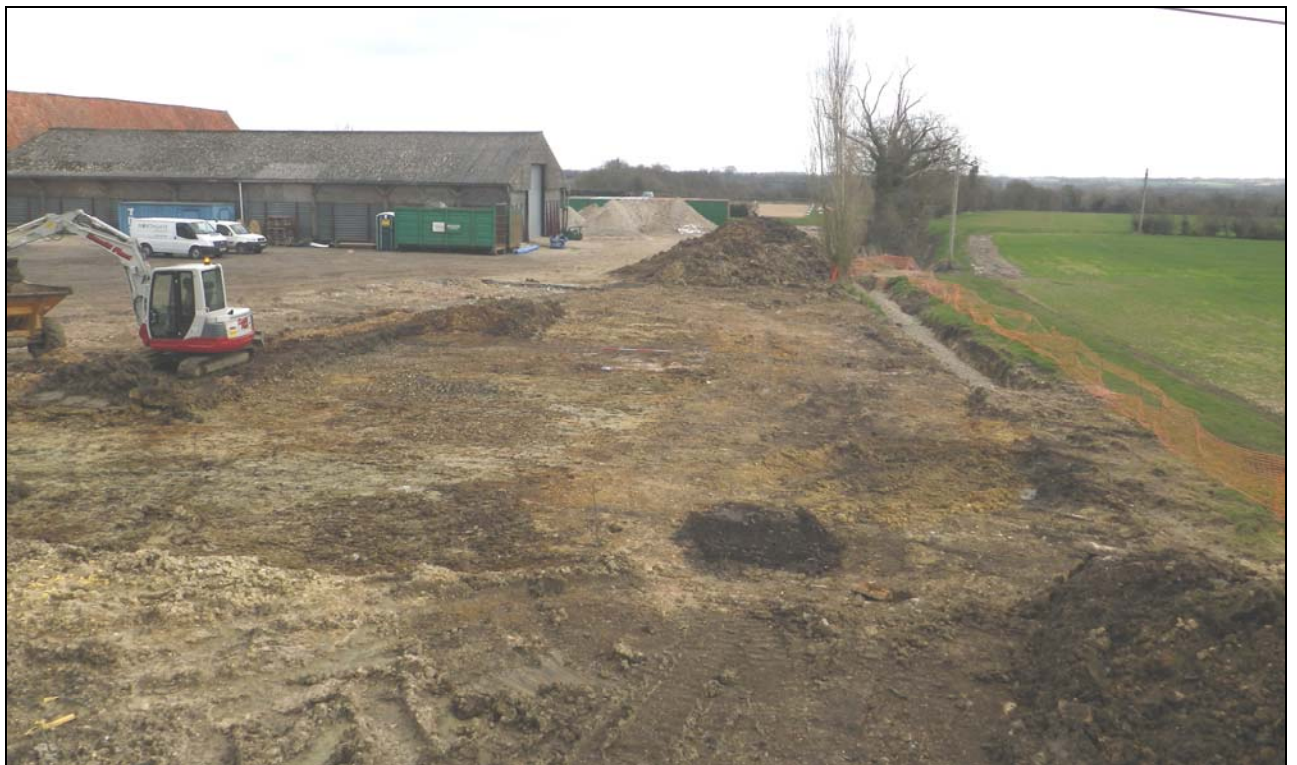
Plate 1 The stripped area taken from the west (2m scale)
