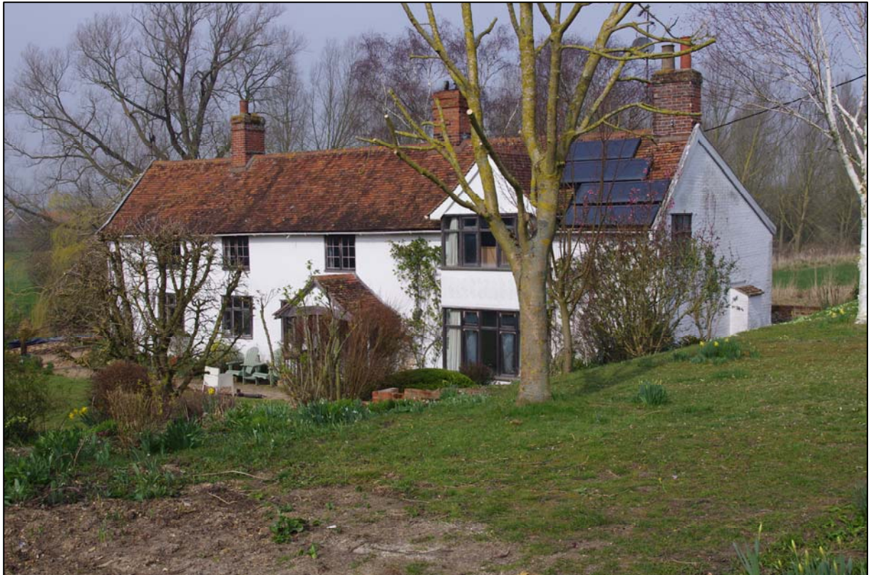
Plate 1. General view Mill House cut into the west facing slope, camera facing NW (ref. HXB 88)
