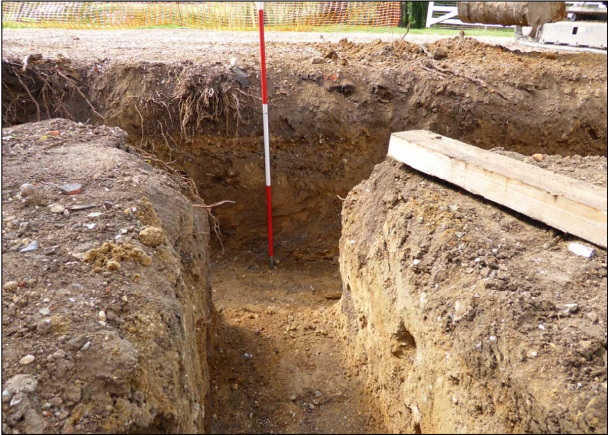
Plate 7. Footing at west end of house showing the abrupt interface between The overburden and the natural subsoil (ref. HXB 90)
