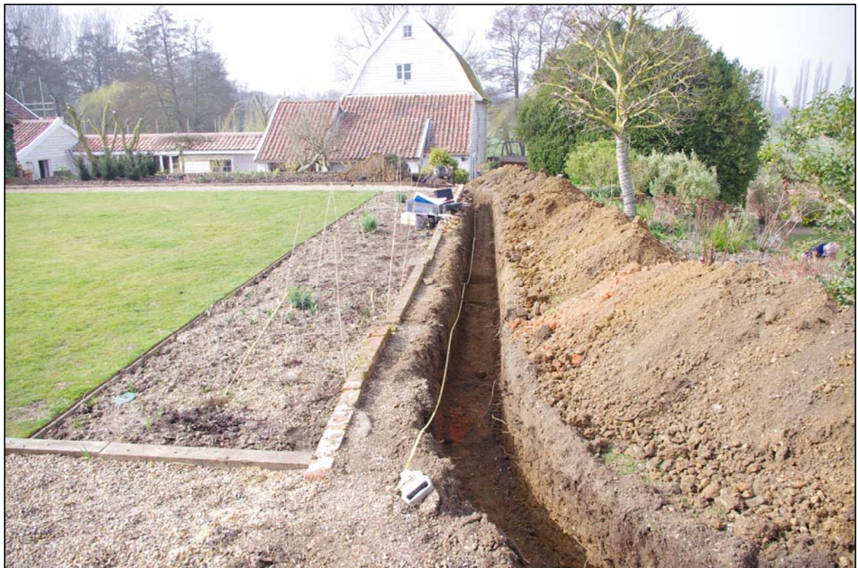
Plate 2. general view of biomass heating duct trench in the vicinity of the grave. The mill building can be seen in the background (ref. HXB 88)
