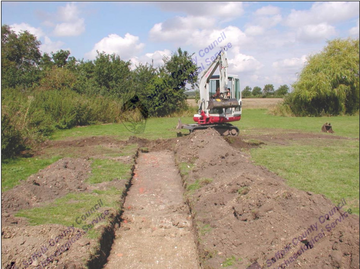
Backfilling Trial-Trenches
