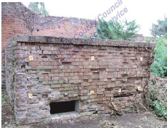
Figure 2. The shelter, south elevation
