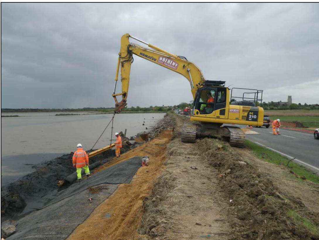
Plate 6. east face of causeway during reconstruction, camera facing south (ref. HWS 41)
