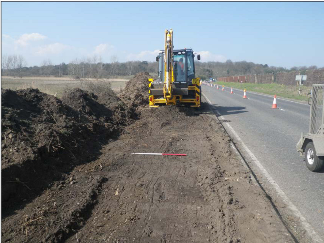
Plate 1. Topsoil strip, western verge, camera facing north (ref. HWS 33)
