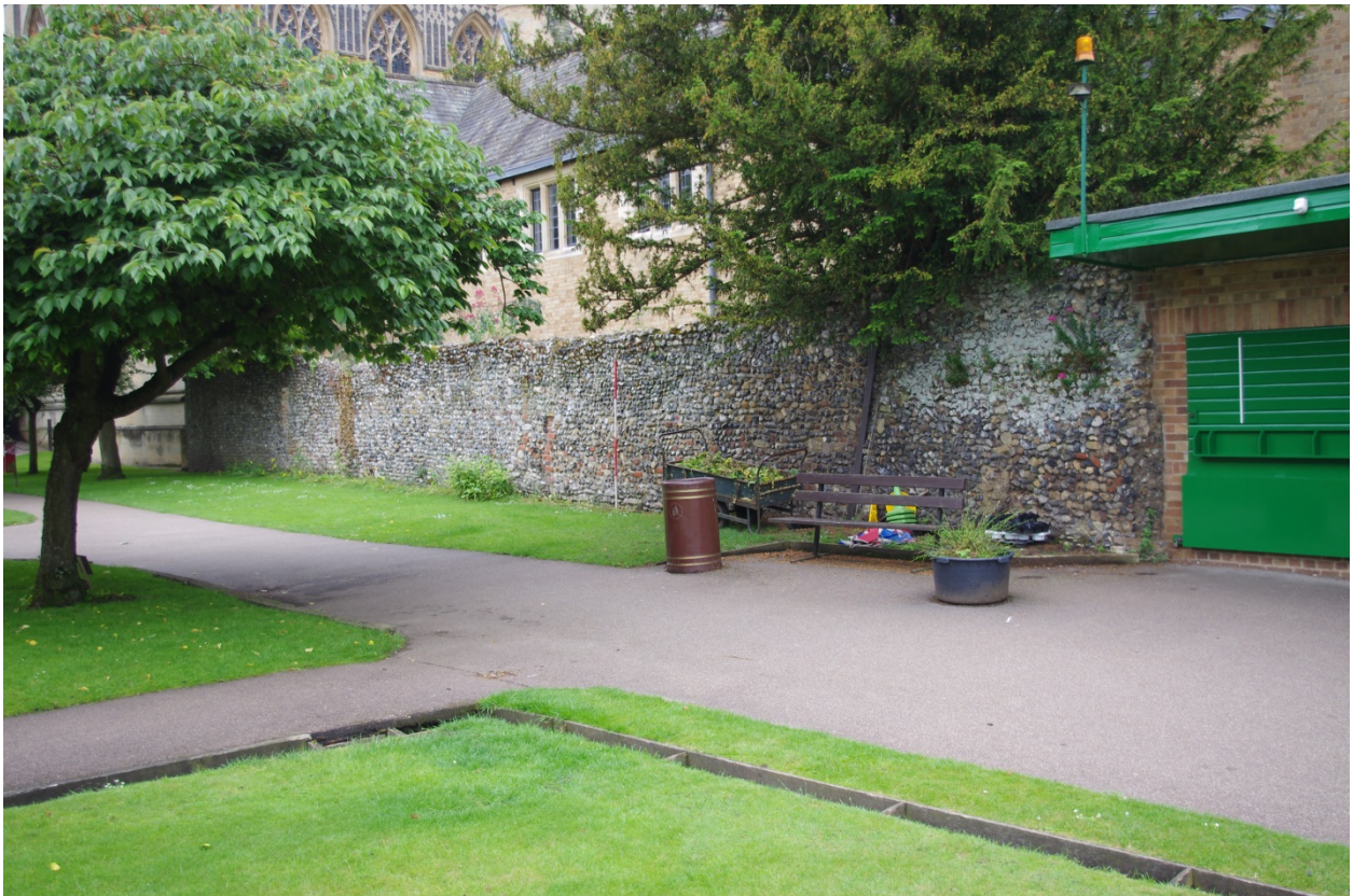
Plate 7. East boundary wall behind the refectory viewed from the east side. The wall from the bowls hut to St James' probably has its origins in the 16th or 17th century with the sections at the far end being rebuilt in the 19th and 20th centuries.
