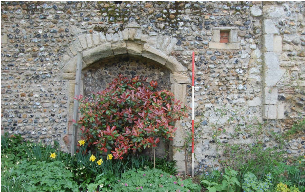
Plate 4. The stones that make up the surveyed door stones are consistent across the top and down the left side and the flint-work to the left is unbroken to the door edge indicating that these are contemporary original features. The top stone of the right jamb is not well matched with the springing point and the absence of the strainer course suggests that this part of the wall has been repaired. The column of stones to the right is the quoin that forms the NW corner of Building 1 - this does not extend to the ground and therefore has also been remodelled.
