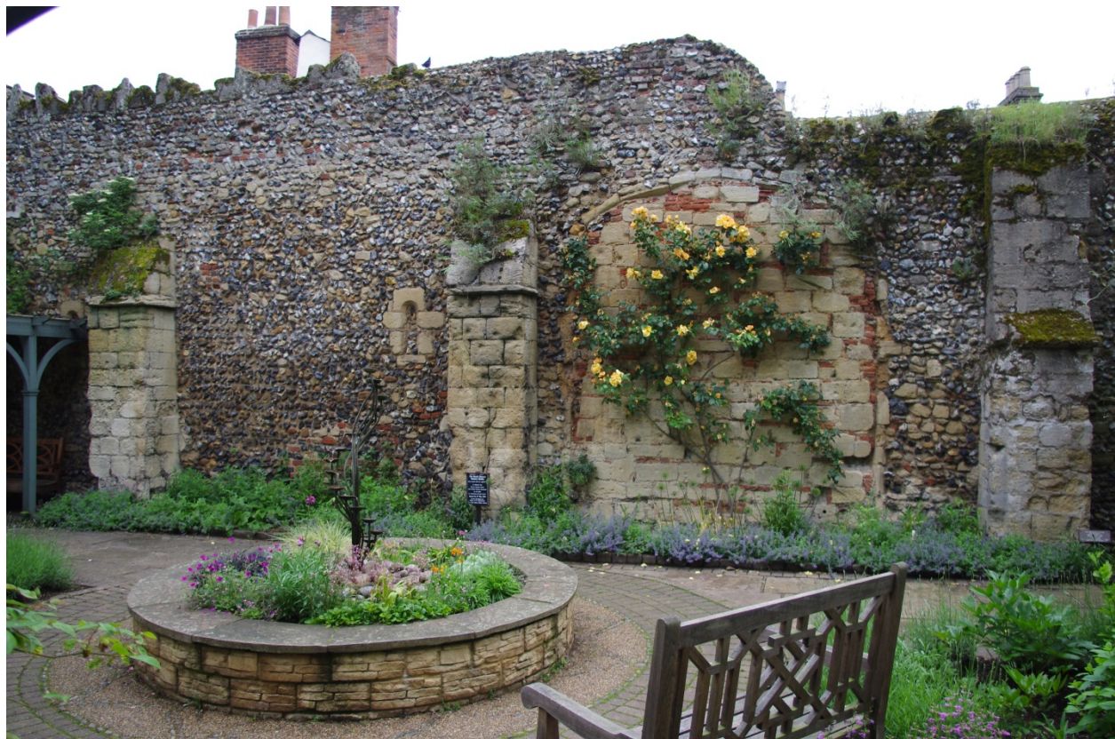
Plate 8. Stable and brew house range on the north side of the great courtyard which were also repaired following the 1327 riots. The wall exhibits pre-riot Norman features (the short buttresses and small window) together with later styles. The arch shape and stones of the large blocked gateway is similar to the surveyed door suggesting that they may be contemporary.
