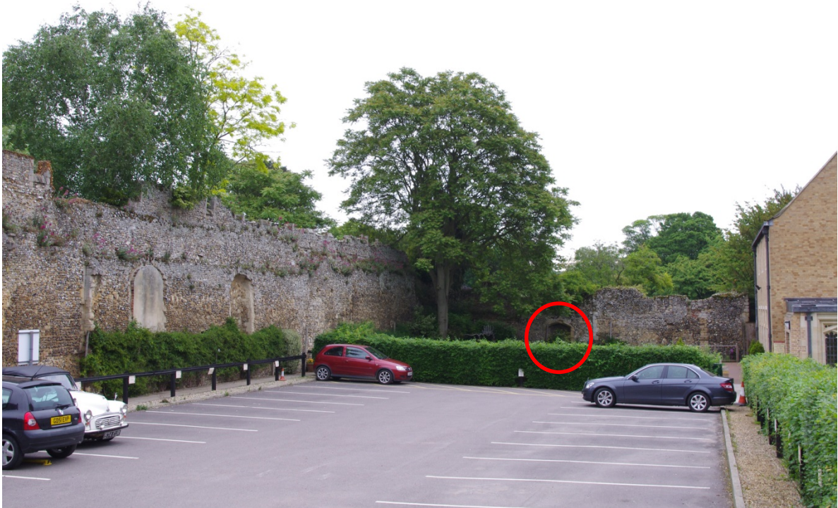
Plate 2. The surveyed door (circled) between the remains of abbey buildings. Immediately to the right of the door is the exterior face of an end gable (Building 1) whilst to the left of the picture the interior face of a second building (Building 2) can be identified by the tall windows. Building 2 stops just beyond the red car and the survey door is set within a length of wall added in the 14th century which joined the remains of the two earlier building together
