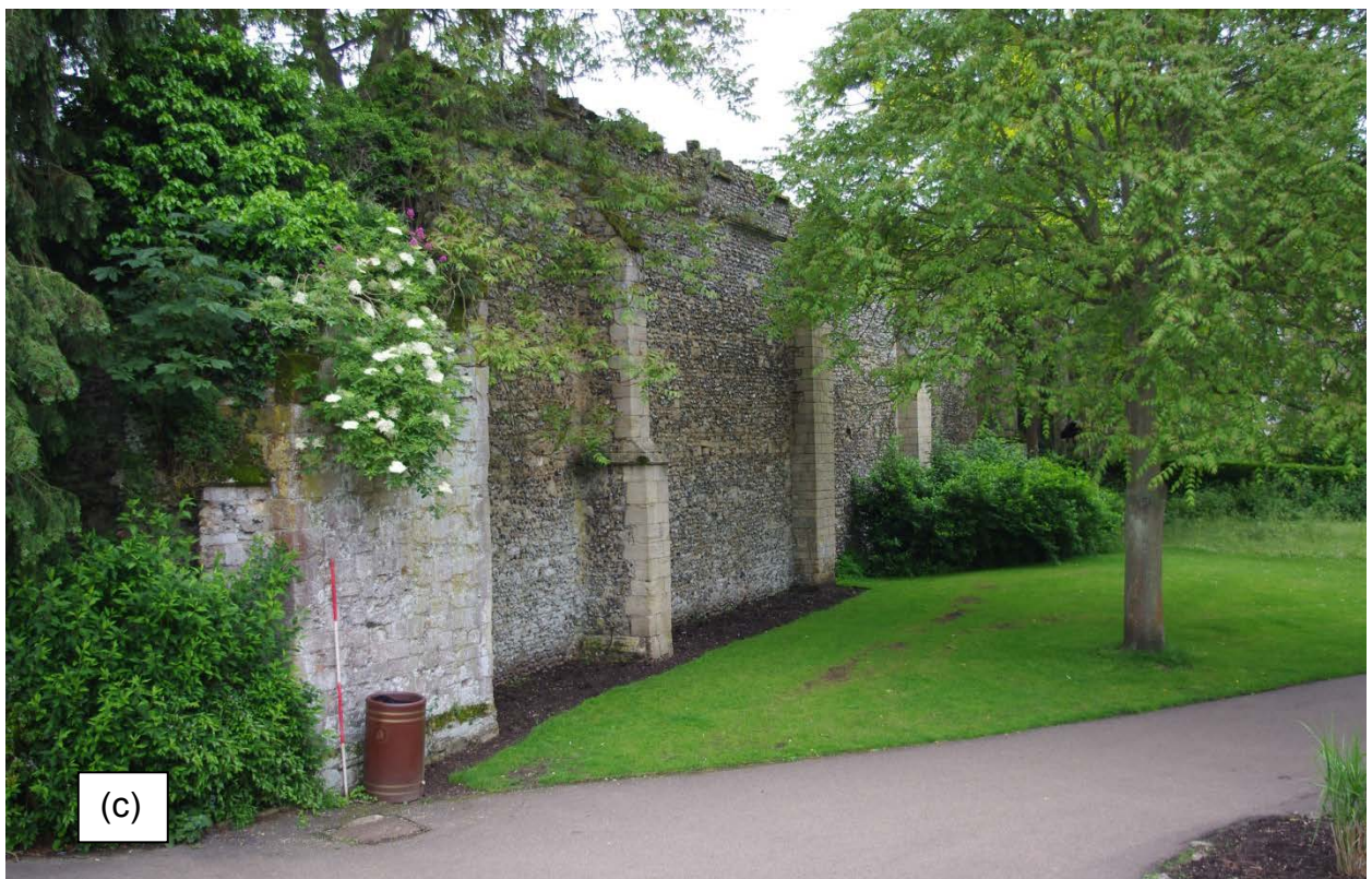
Plate 6. The north wall of the Precinct Yard was extended westward to join with the precinct wall and eastward to form the current corner in the 14th century (c). The limit of the original 12th century building is defined by the flat buttress at the far end of the narrow bed. The features of the later building include the bay (behind the bin) beneath what would have been an oriel window at first floor level and later buttressing on the corner and north wall face. The blocked window (6a) and door (6b) are occur with the early section of the walling but the door certainly is a post 12th century inserted feature.
