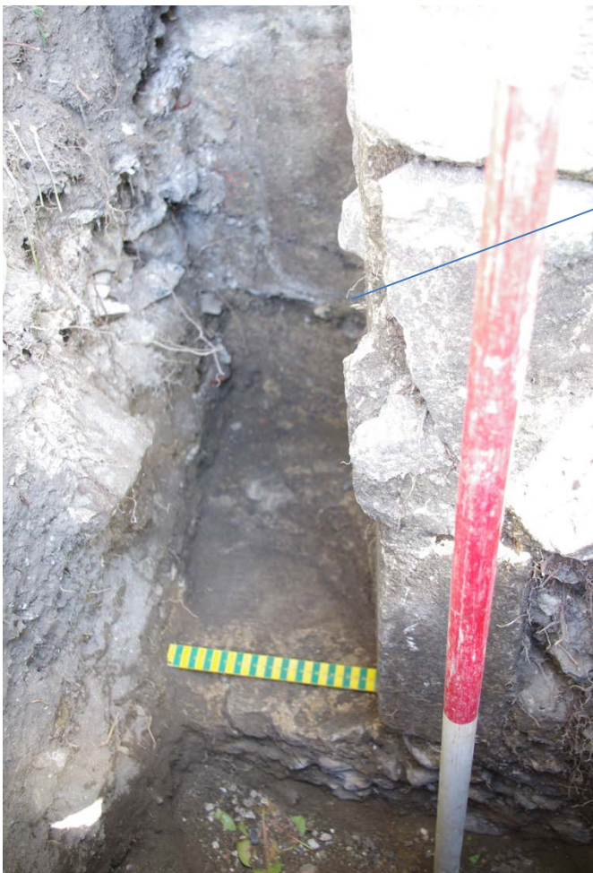
Plate 4. The stones that make up the surveyed door stones are consistent across the top and down the left side and the flint-work to the left is unbroken to the door edge indicating that these are contemporary original features. The top stone of the right jamb is not well matched with the springing point and the absence of the strainer course suggests that this part of the wall has been repaired. The column of stones to the right is the quoin that forms the NW corner of Building 1 - this does not extend to the ground and therefore has also been remodelled.
