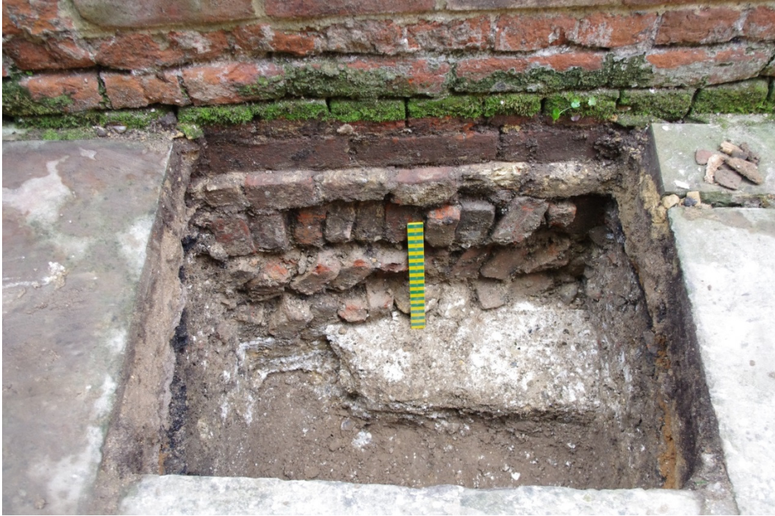
Plate 7. Test hole 5 showing the 'loose-laid' brick foundation of the detached kitchen overlying an imported layer of rammed chalk, possibly the floor of the medieval kitchen which once stood on this spot. The chalk was laid over a buried topsoil (the brown soil at the bottom of the excavation) which produced a group of pottery that is dated to no later than the 14th century. The scale is 0.3m.
