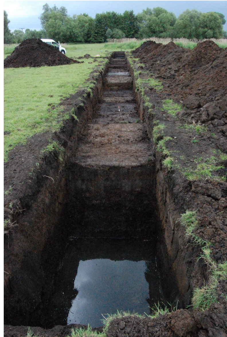
Plate 4. Trench 02, facing northeast
