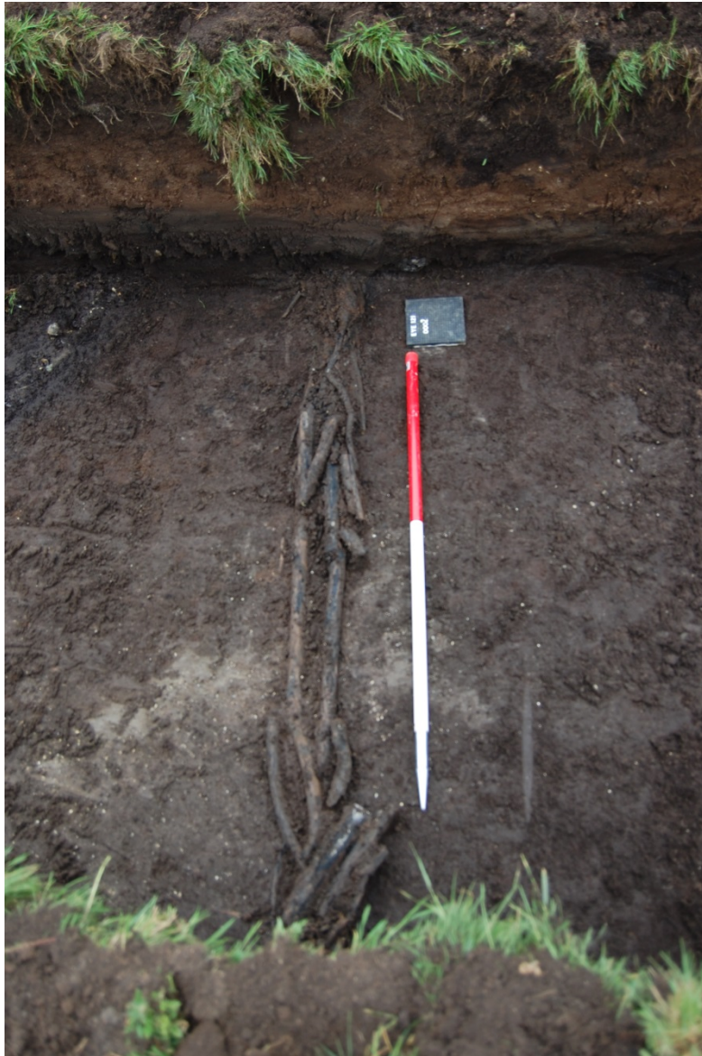
Plate 3. 0002 faggott drain, facing south-west (1m scale)
