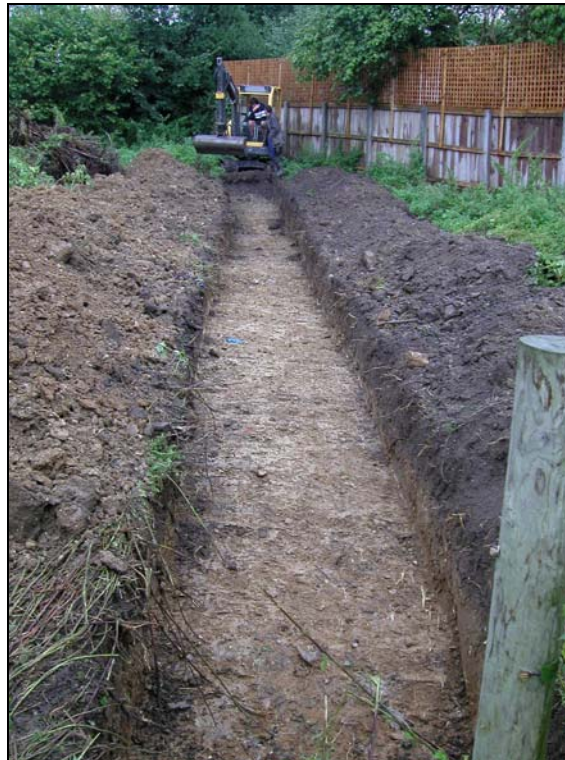
Trench 2 upon completion
