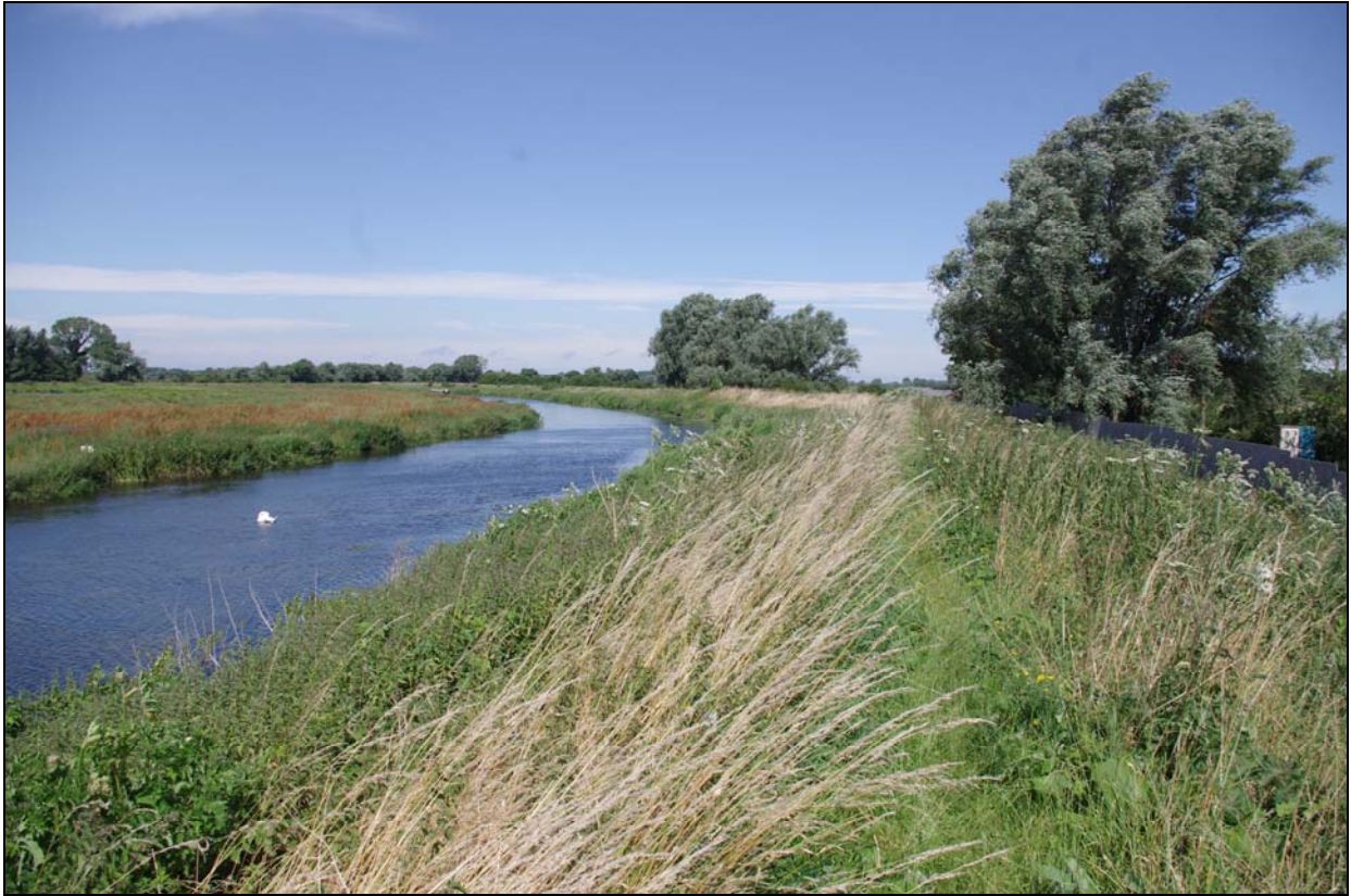
Plate 1. River Lark, overlooking site (facing WNW)
