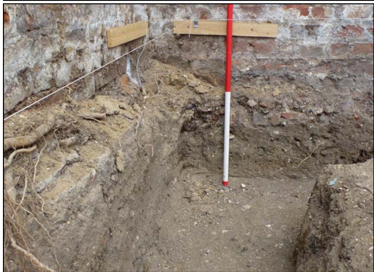
Plate 2. Stratigraphy revealed after excavation of the ground beam trench
