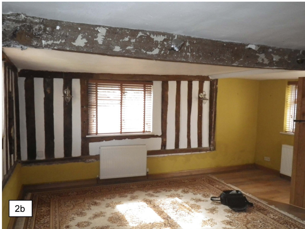
Plate 2 a) and b). Close-studding with concealed braces at the eastern end of the house which probably dates to 16th century. Inserted timbers and a crudely lap-jointed sill beam, to the left of the ceiling bridging beam (top), are the result of later modification. The limit of the framing (bottom) shows the original south east corner and line of the rear wall. The windows and ceiling retain their original positions.
