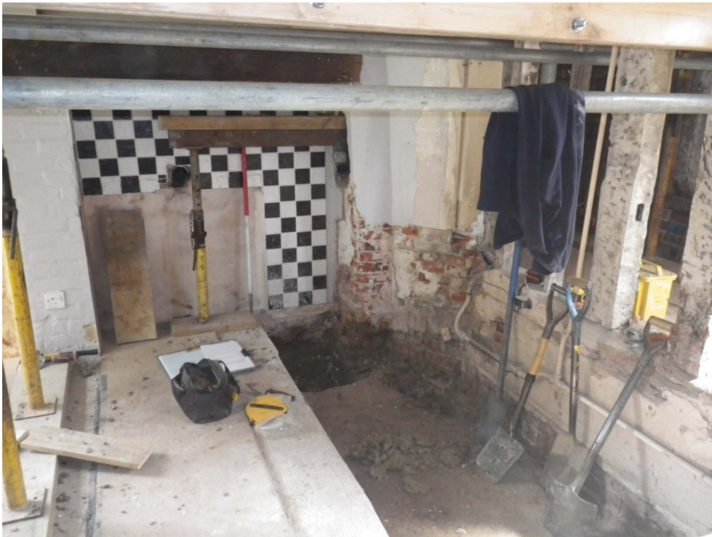
Plate 3. The kitchen of Street Farmhouse with the floor partly excavated. The fireplace probably dates from the 18th century but was greatly altered in the 19th and 20th century. The chimney has been fitted into a narrow chimney bay but partially envelopes the bridging beams that span the width of the house suggesting that this is a replacement stack. The original back wall of the house (behind the shovels) has been underpinned with brick and concrete in the relatively recent past.
