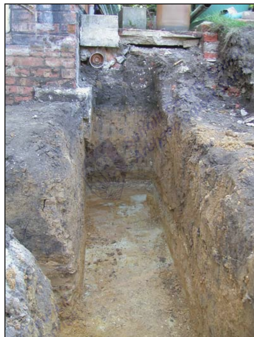
Plate I: View of footing trench - facing south
