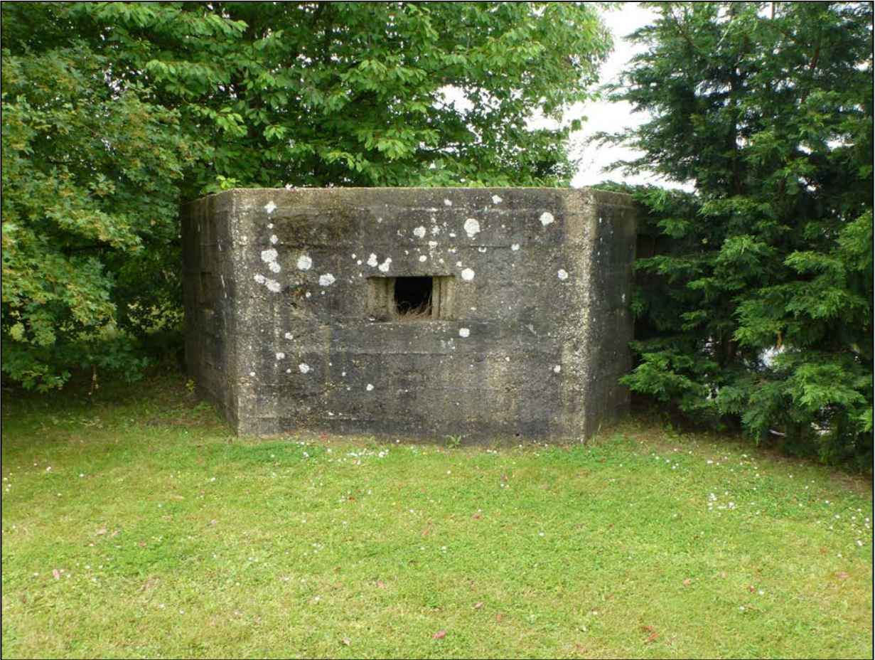
Plate 5. Pill-box in southern corner of development area, camera facing south (ref. HWZ 39)
