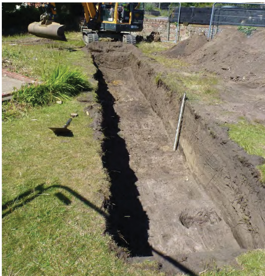
Plate 1. Trench 1, camera facing northwest (ref. HWZ 40)
