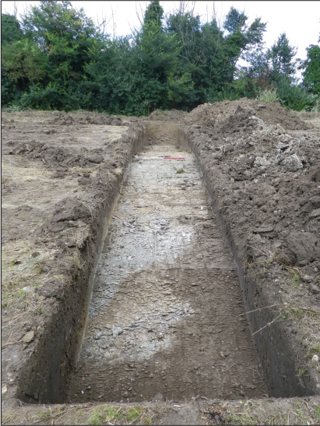
Plate 1. Trench 2, looking N
