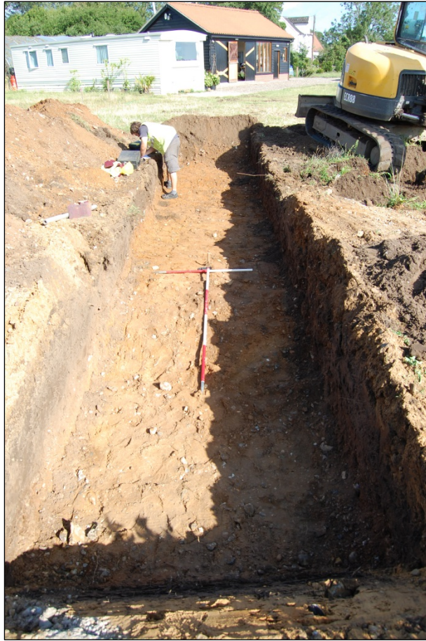
Plate 1. Trench 1 plan, looking north-west. 2m vertical and 1m horizontal scales.
