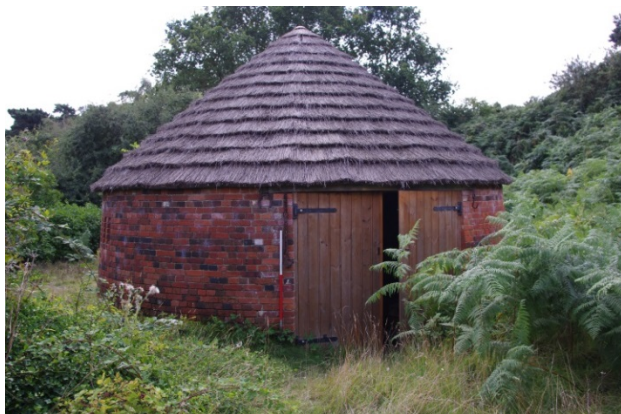
Plate 2. View of the kiln looking south, showing new roof and double-doors (1m scale)
