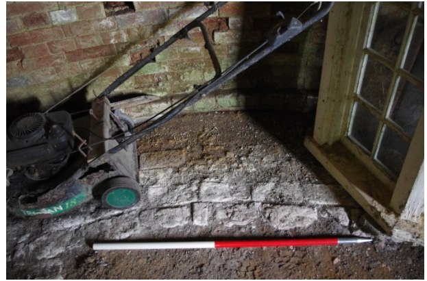
Plate 5. Detail of floor bricks with off-set red brick course above (1m scale)
