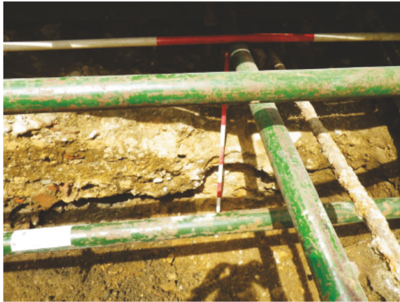
Plate 2 Detail looking north at wall 0004 showing through wall 0001, 1m and 2m scales.
