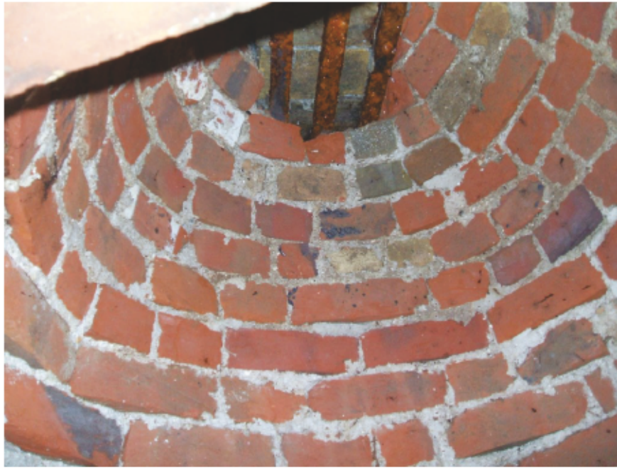
Plate 6. Inside the well (see pl.5) cap
