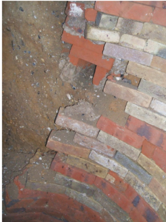
Plate 5. Probable 19th century well on the south side of Hole 2 (this unbonded wall later collapsed), a cemented red brick insertion can be seen in the centre of the photograph, which may have been an inlet for a soak away.
