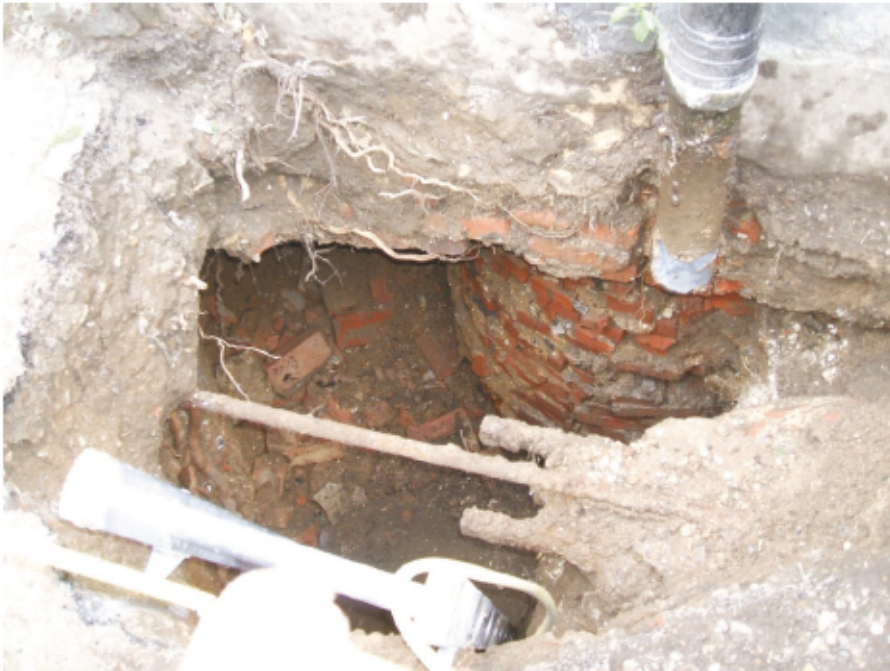
Plate 5. Showing a probable well, c.18th century, under Abbey House and beneath an internal partition between two separate elements of the building.
