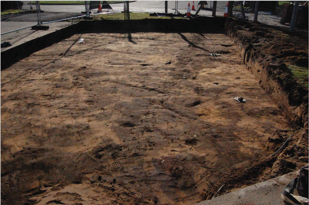
Plate 1. Site after machine stripping, prior to removal of layer 0001 (facing south-south-west)
