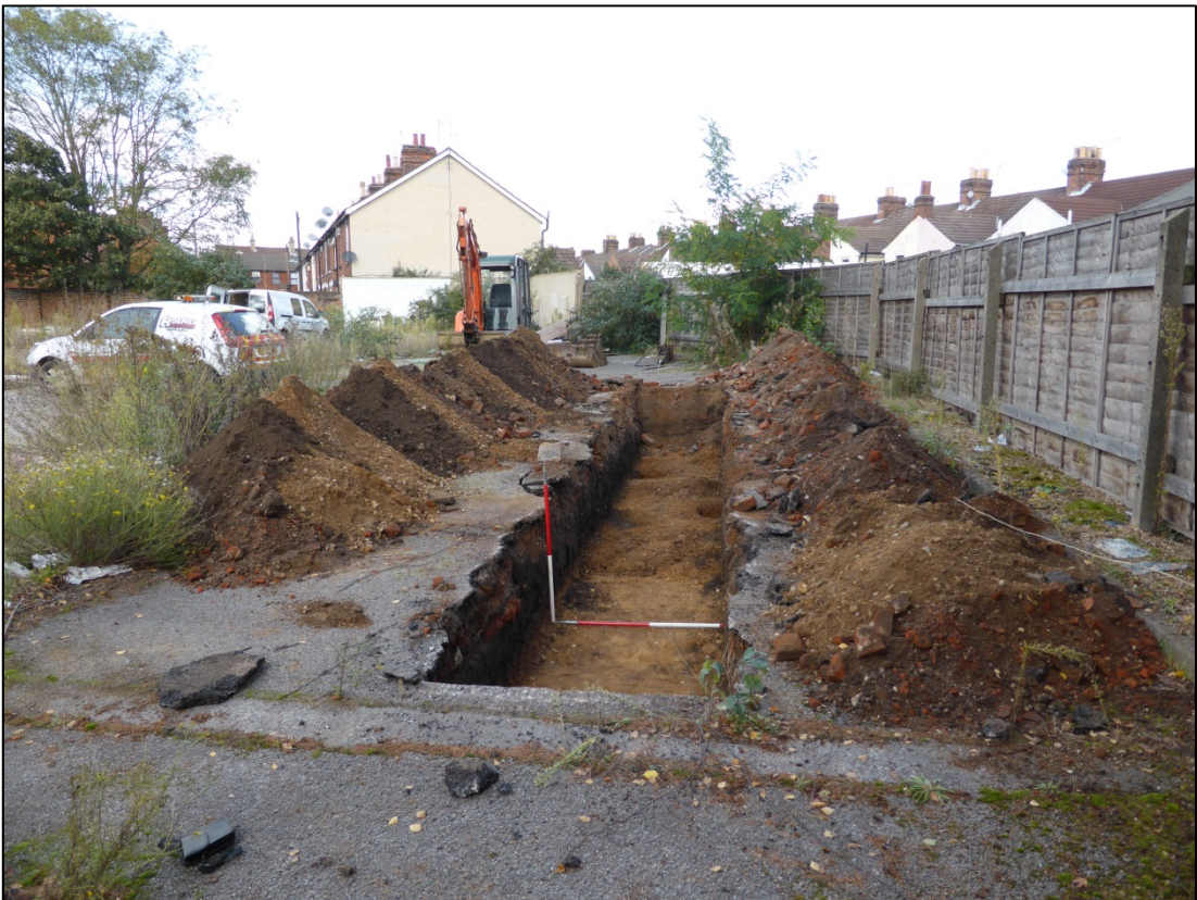
Plate 8. General view of Trench 3, camera facing north (ref. HWS 88)
