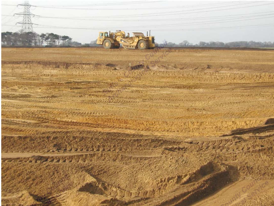
Figure 1: View across the site showing soil stripping in progress
