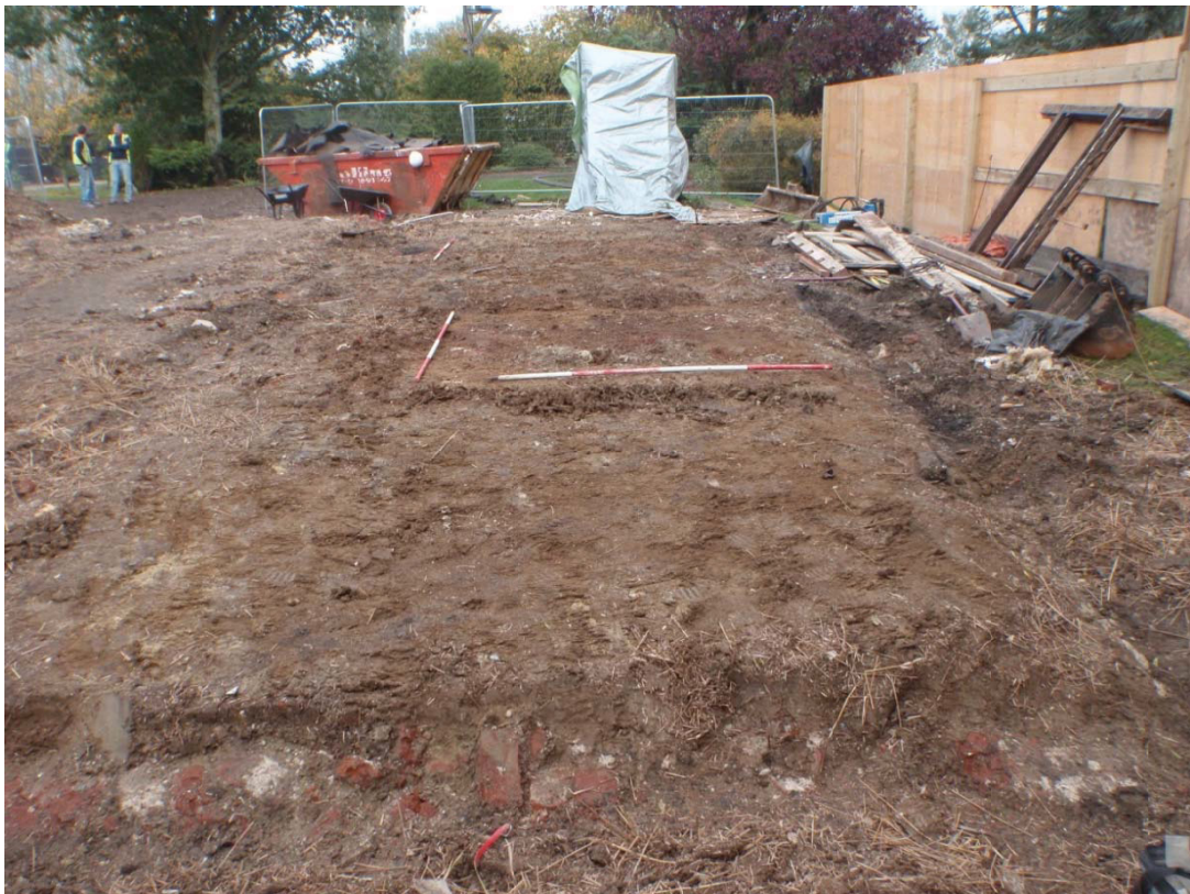
Plate 2. The site of the north-south wing following the dismantling of the frame looking north. The building has been demolished to the original 16th century floor level; underpinning of the timber sole plate with brick (foreground) during the 19th century necessitated the lower of the surrounding external ground, creating the effect that the internal floor area is raised.
