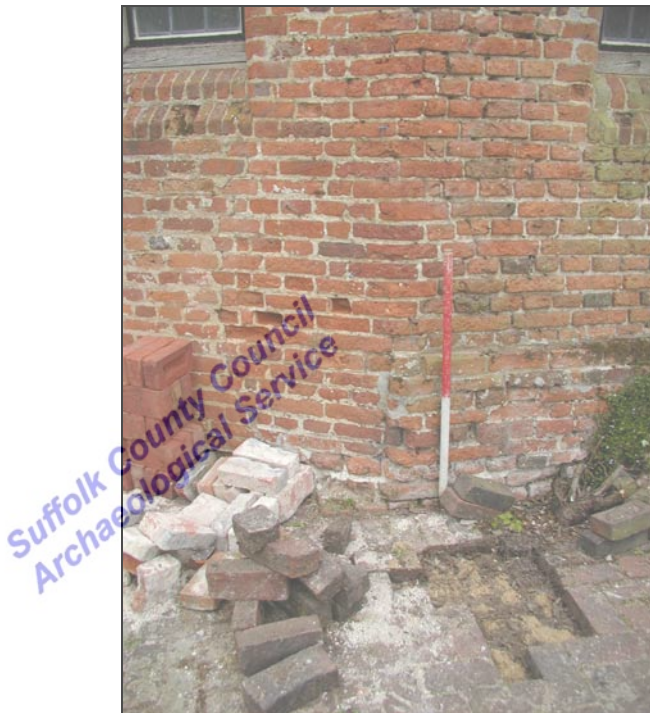
Plate 29 Diagonal wall, truncated plinth
