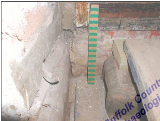
Plate 15 Wall 0007 butting against 0011
