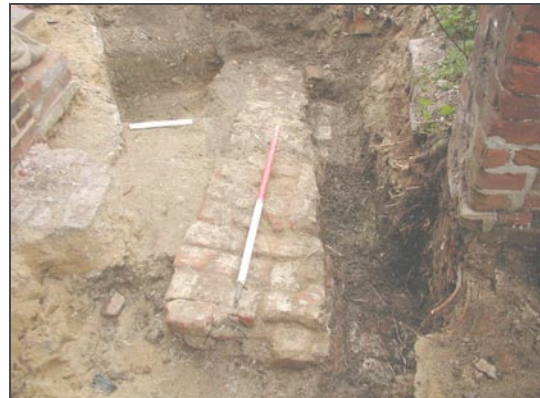
Plate 4 Trench 2; wall 0029 from the west
