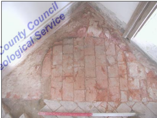
Plate 23 Base of fireplace 0041
