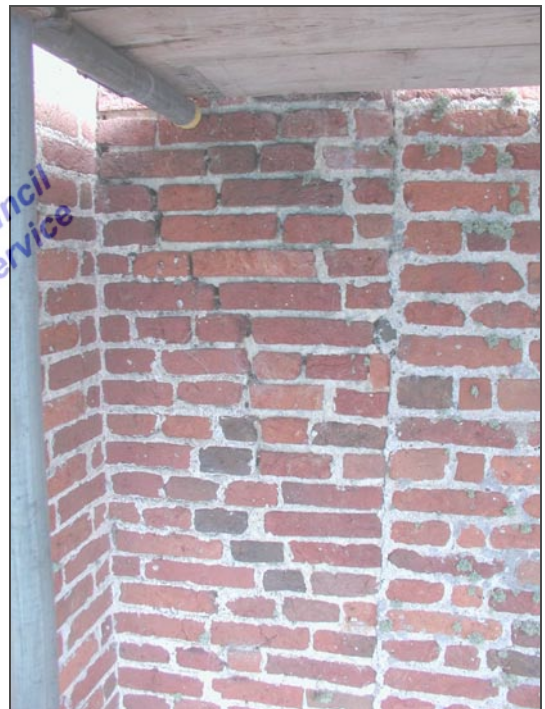
Plate 16 Wall 0010; truncated diaper work
