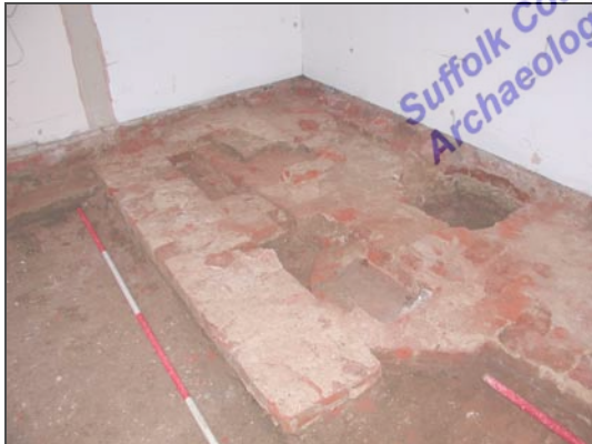
Plate 21 Detail of wall 0005 & 0009
