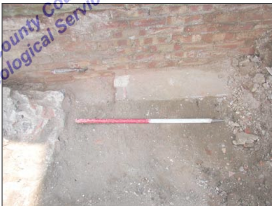
Plate 45 Concrete footing for wall 0075
