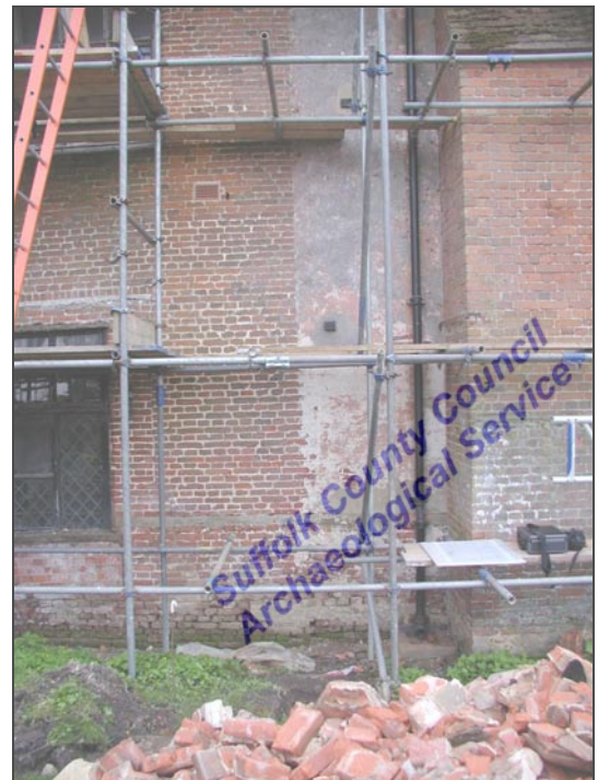
Plate 11 Straight junction in render
