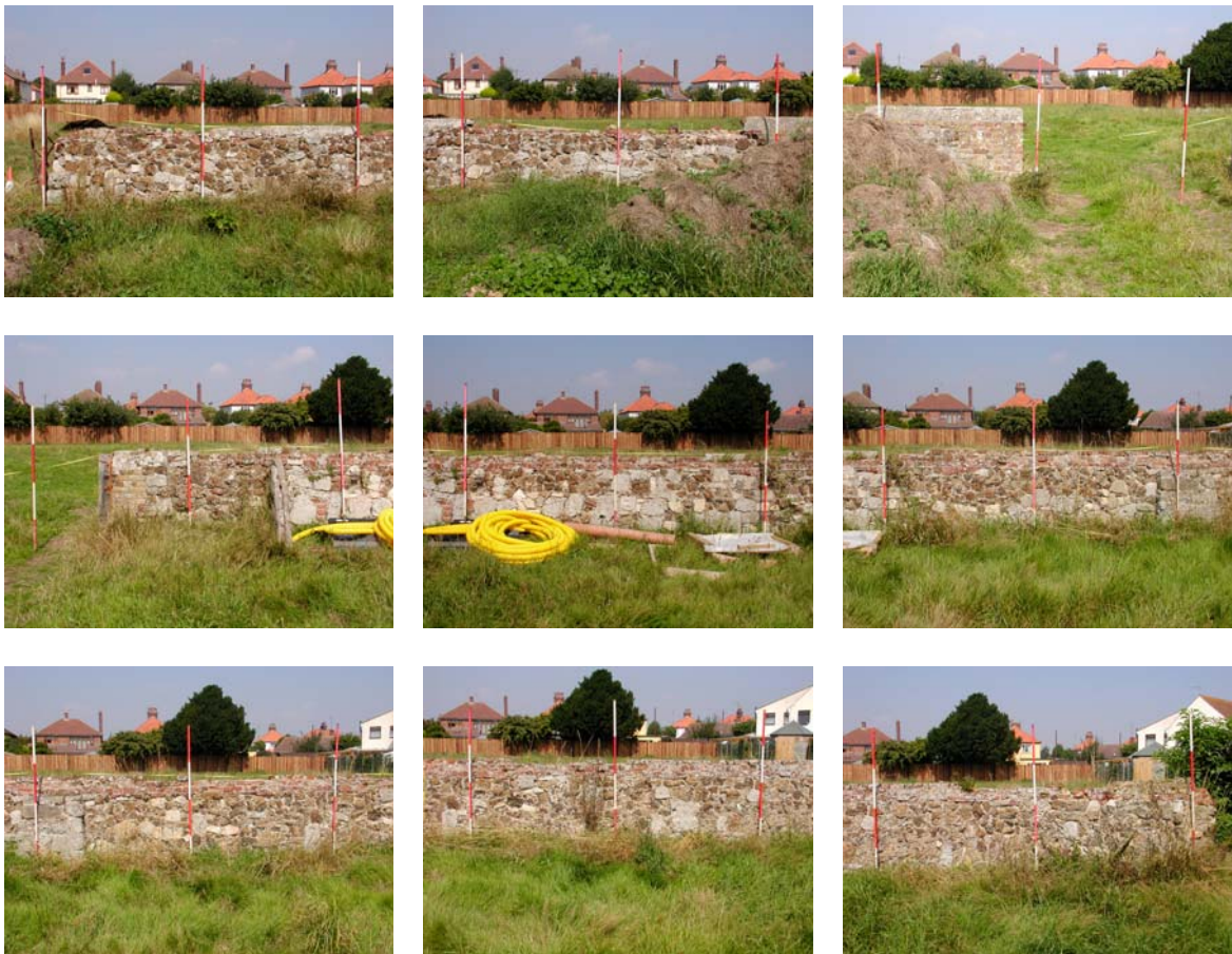
Plates II-X: South Face of Wall
