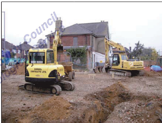
Plate II: excavations for groundbeams underway (7 th November 2006)
