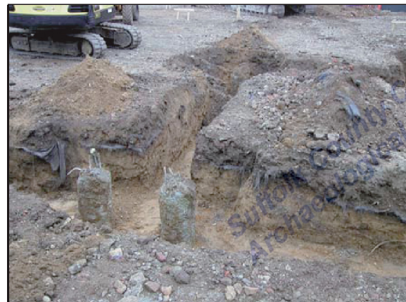
excavated groundbeam trench (7 th November 2006)
