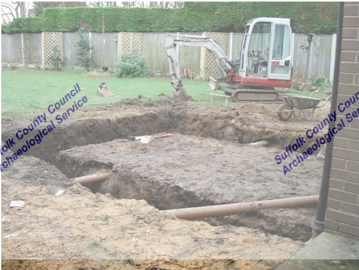
General View of the site (looking south-east)
