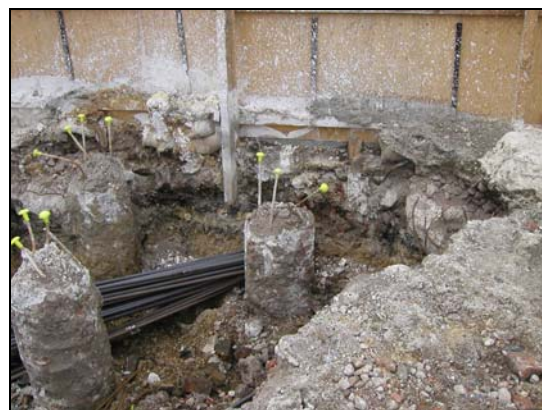
Plate II: Pile Cap Against SW boundary View facing SE
