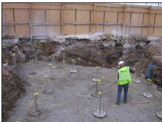
Plate I: Pile Cap Against SW boundary View facing SE
