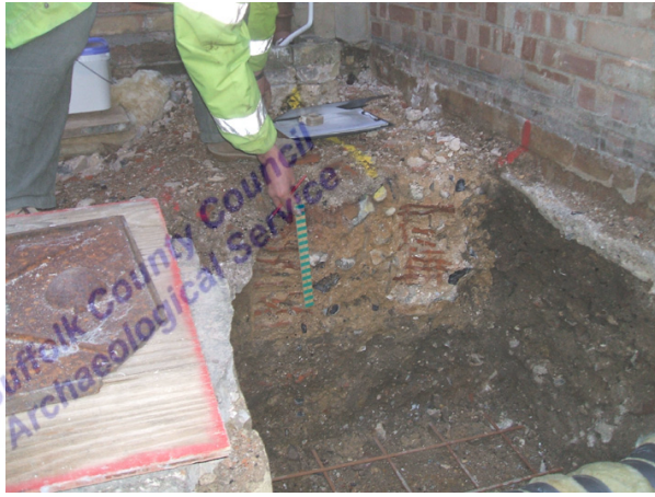
Figure 3. Cross section of flint wall
