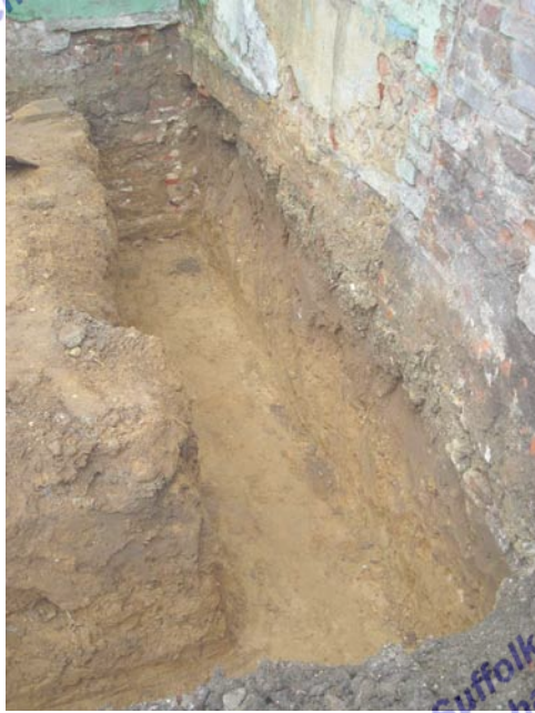
Plate 1: A section of excavated footing
