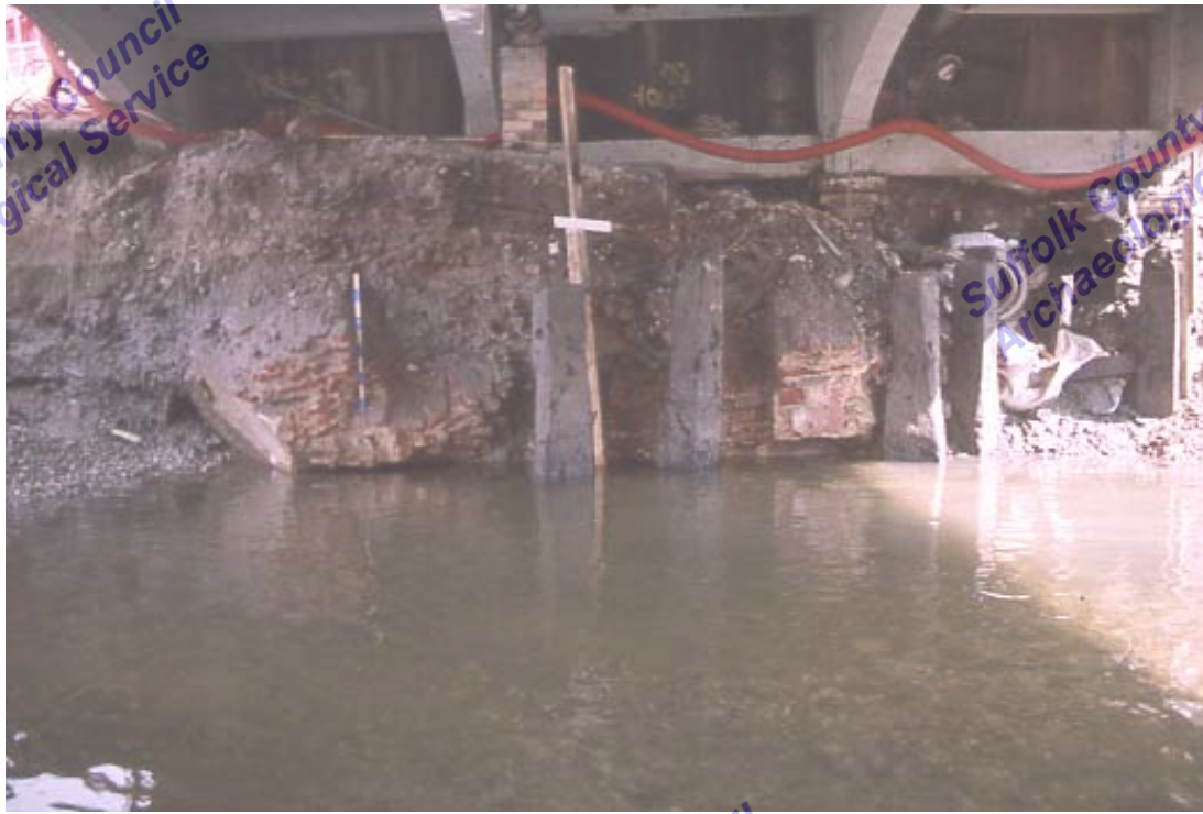
Figure 17. Cross-section of the brick bridge, 0054, behind timber pile of the later bridge
