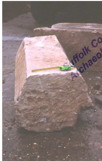
Figure 12. Voussoir part of an arch ring
