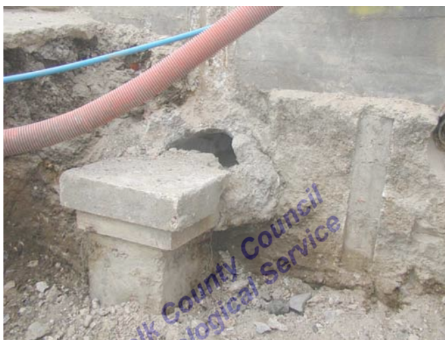
Figure 28. Explosive holes behind the piers
