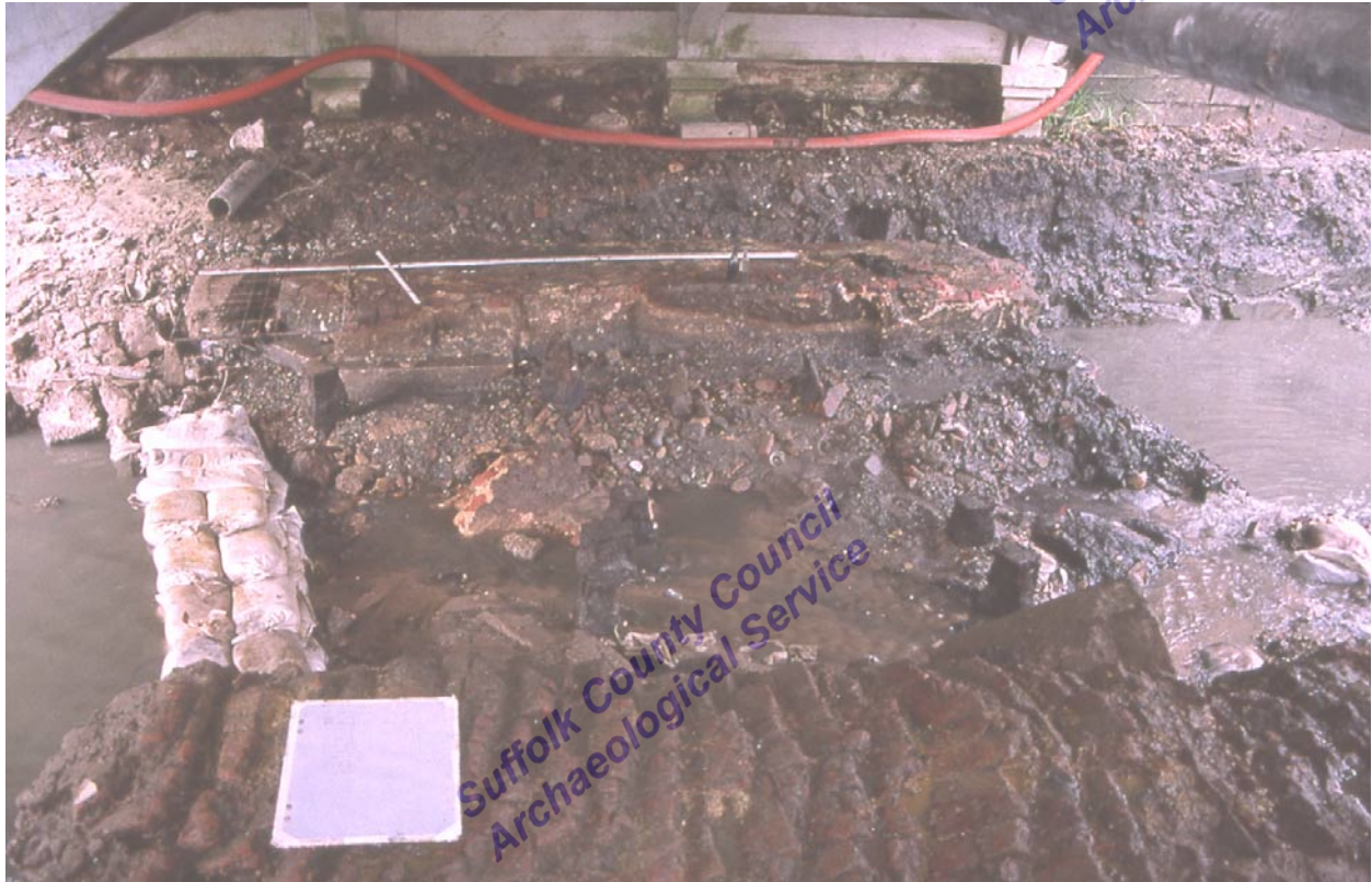
Figure 14. Piers 0101 and 0102. Slump of pier 0102 evidenced by the angled brick courses in foreground
