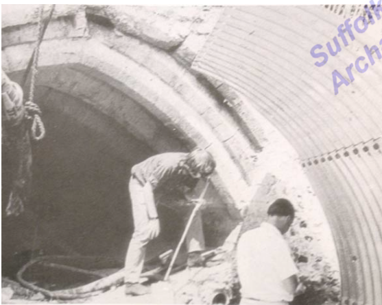
Figure 25. Southgate Street bridge
