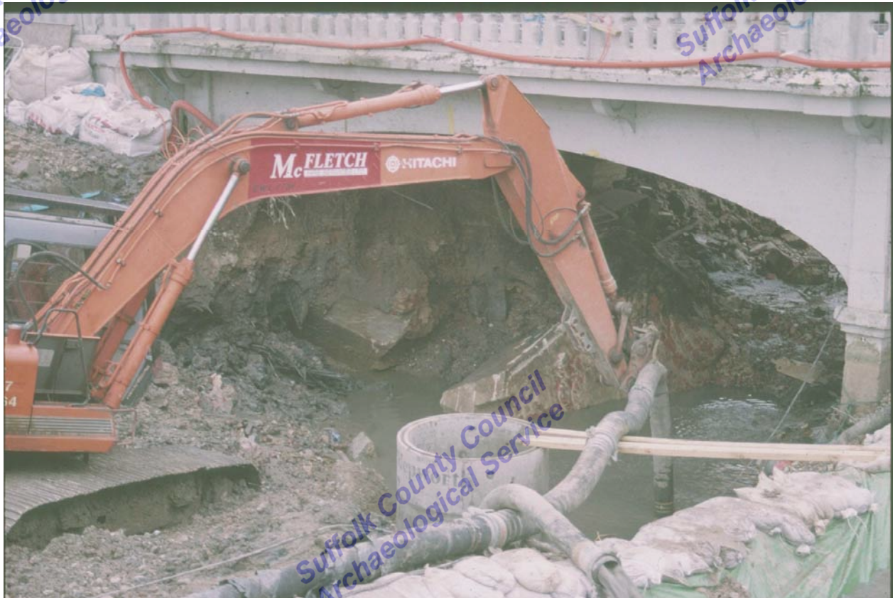
Figure 11. Remains of the brick bridge being excavated adjacent to the Sudbury bank
