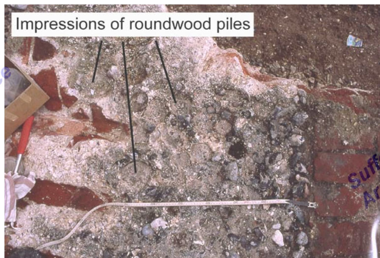
Figure 15. Underside of pier 0101 showing impressions of piles
